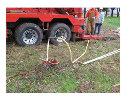
Subject: Tremie-grouting at well New 50 East, showing installed tremie pipe and fitting/hose for grout pumping from rig.
