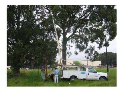
Subject: Removing submersible pump and pipe riser piping from Final Recharge Well.
