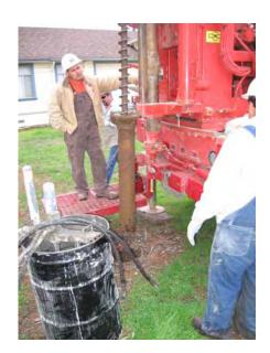
Subject: Overdrilling well New 100 South, showing upper 5' of casing that was pulled from the hole by the augers.
