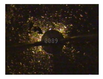
Subject: Downhole video camera survey at "Original Recharge Well" – downward view at 89' depth, showing sediment beginning.
