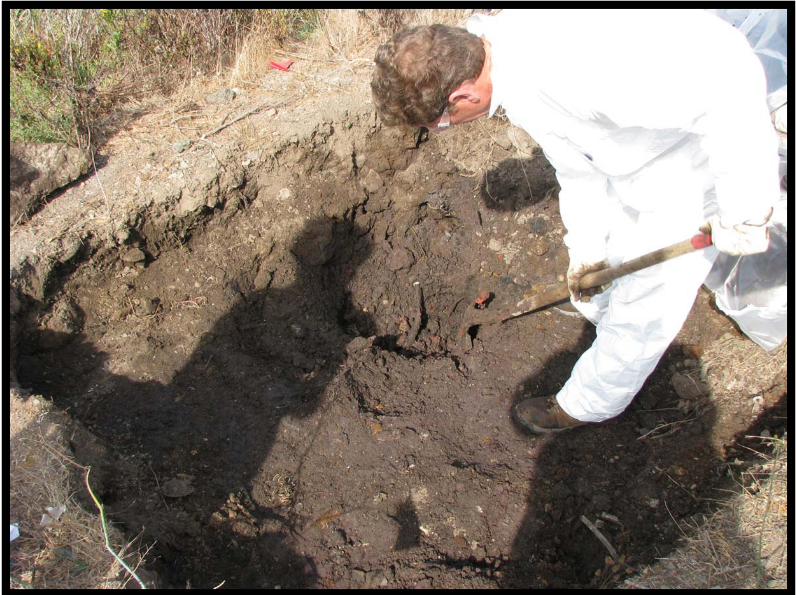
Picture 11. Extent of excavation, Campfire Area II
