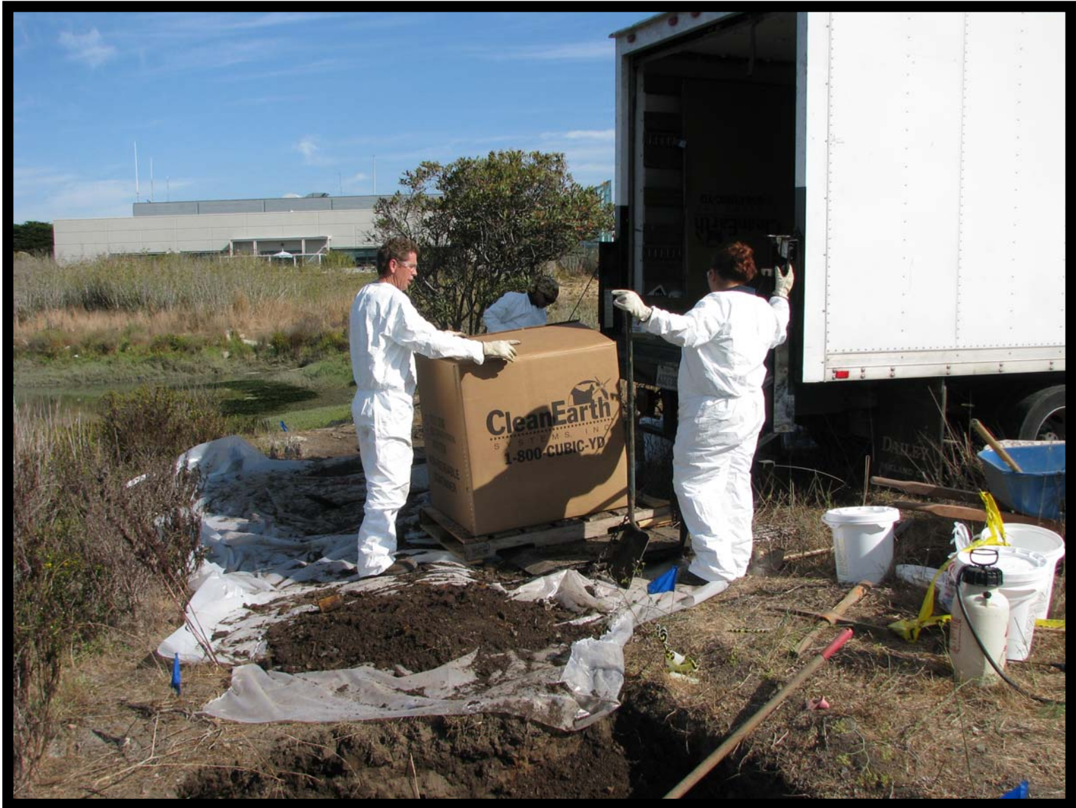
Picture 12. Loading excavated material onto truck
