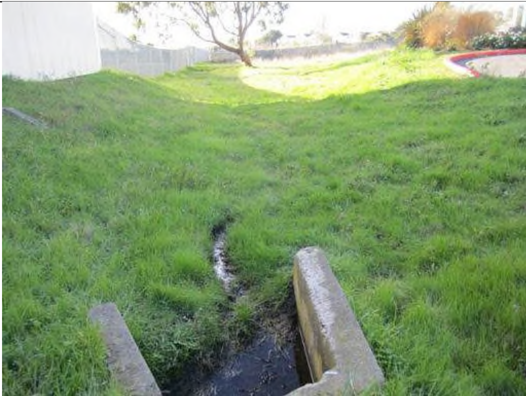
Photo 4. Wetland swale from Photo 3 continues to flow as a channel to the fence line (facing south).
