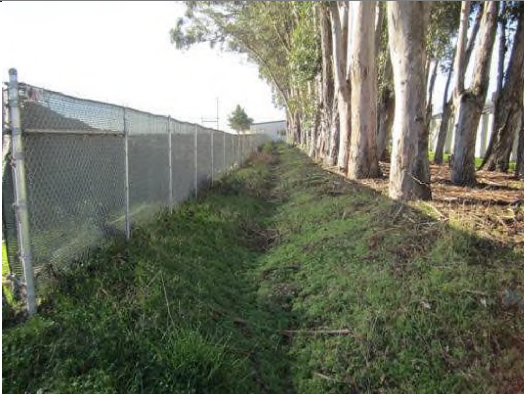
Photo 1. Drainage channel that flows south parallel to Building 275 (facing south).
