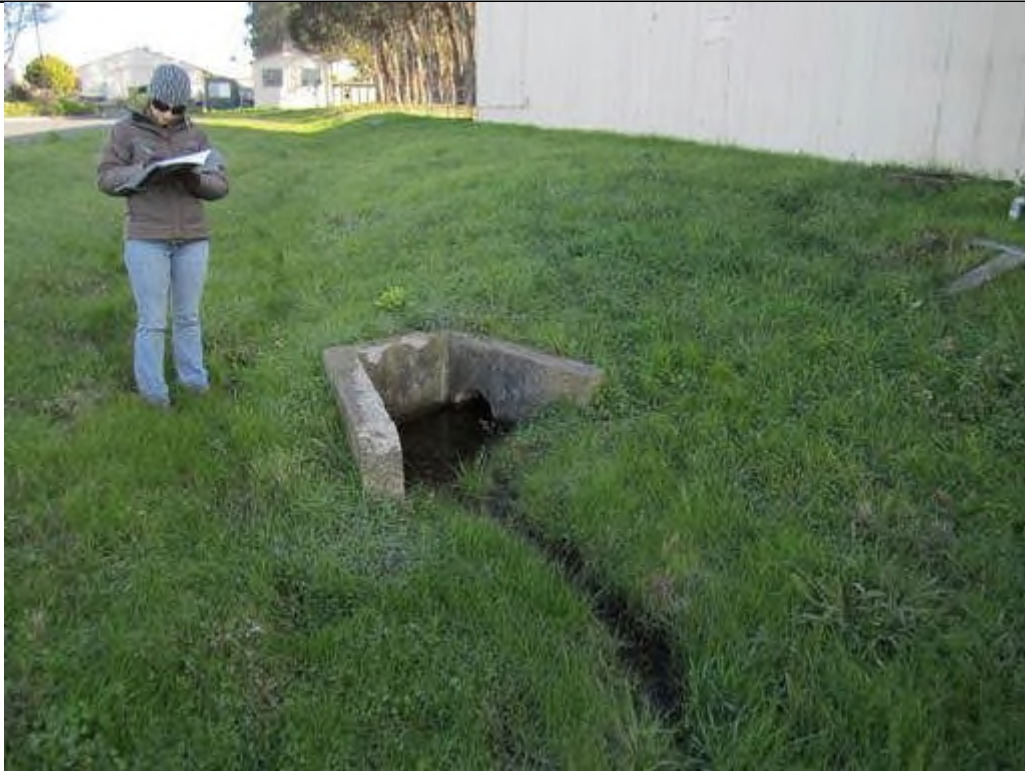
Photo 3. Box culvert west of Building 128. Channel flows underground from previous culvert and exits here where it combines with wetland swale (facing north).
