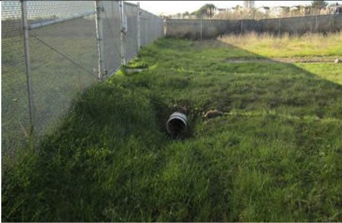
Photo 5. Wetland swale from previous photo flows into a culvert to pass under Heron Drive and continues as a narrow channel (facing south).
