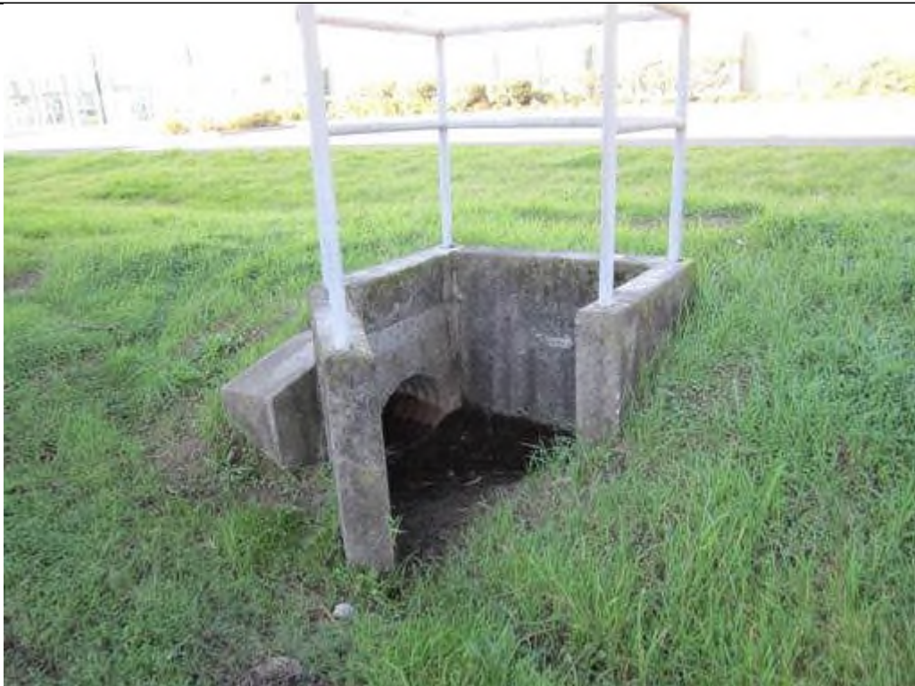
Photo 2. Drainage shown in Photo 1, as it turns west at Building 128 and flows into a box culvert (facing west).
