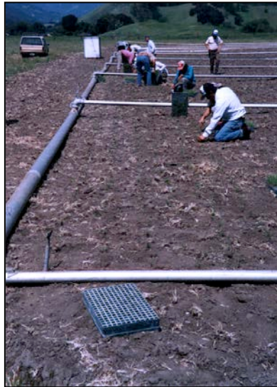
Figure 10. An example of temporary irrigation pipes and sprinklers for establishing plant material in prepared soil.
