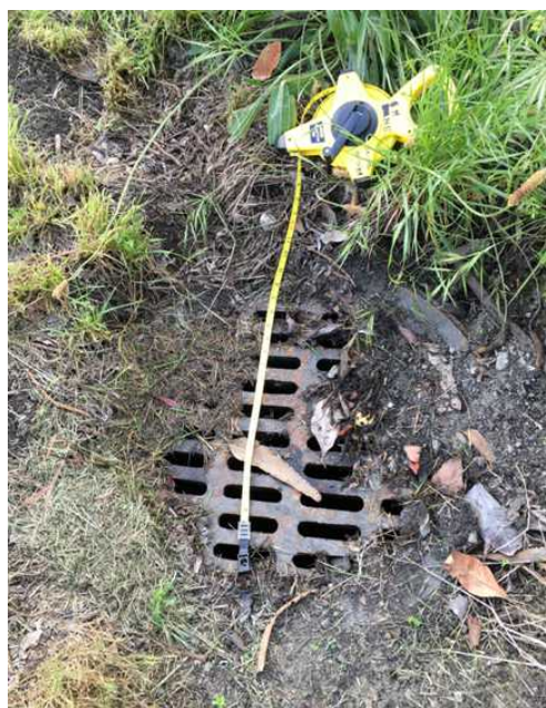
EPA NE Storm Drain, 2-Foot Diameter
