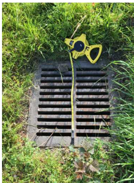
EPA NW Storm Drain, Approximately 2 x 2 Feet
