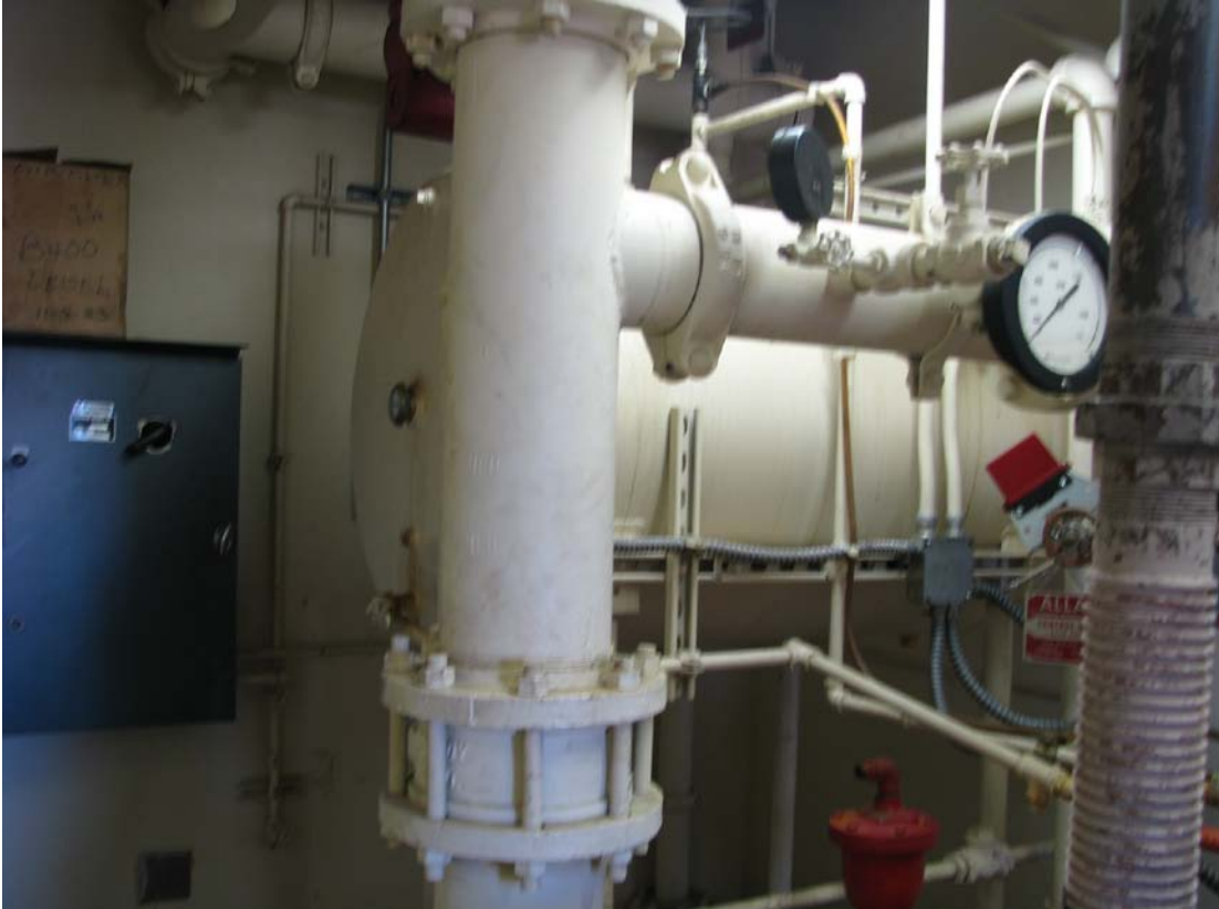
Tanks A-18-5 – Bldg 400
