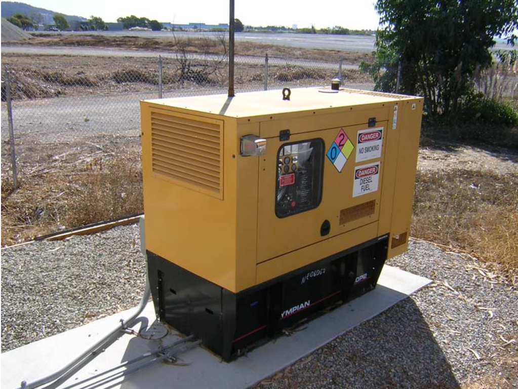
Tank A-18-6 – Outside Bldg 194
