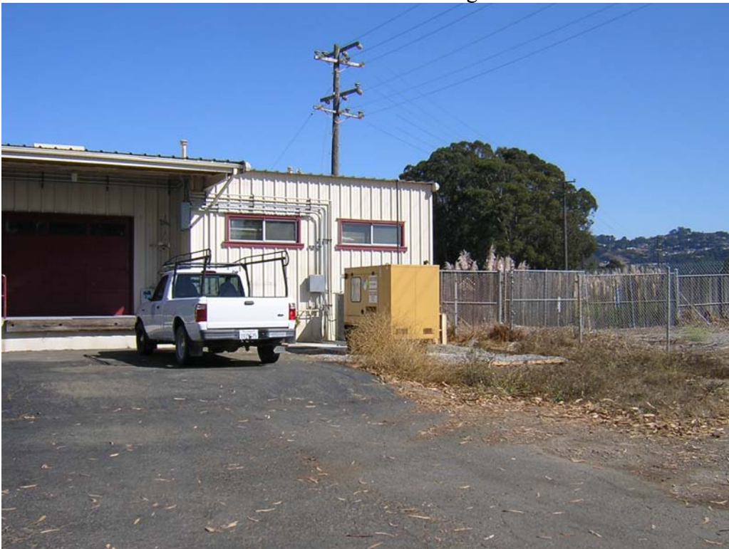
Tank A-18-6 – Outside Bldg 194
