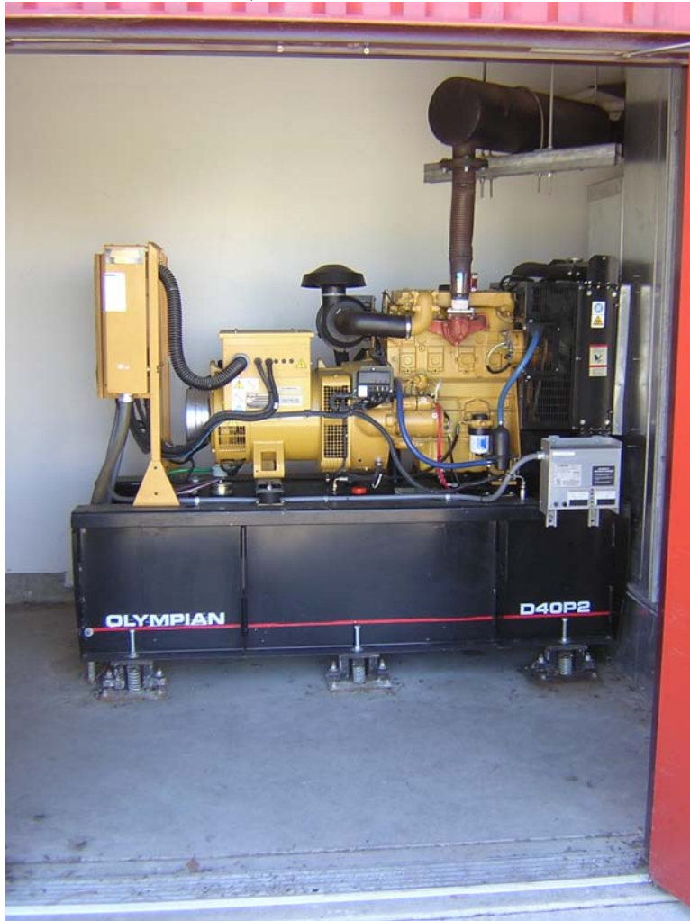
Tank A-18-7 – Bldg 400
