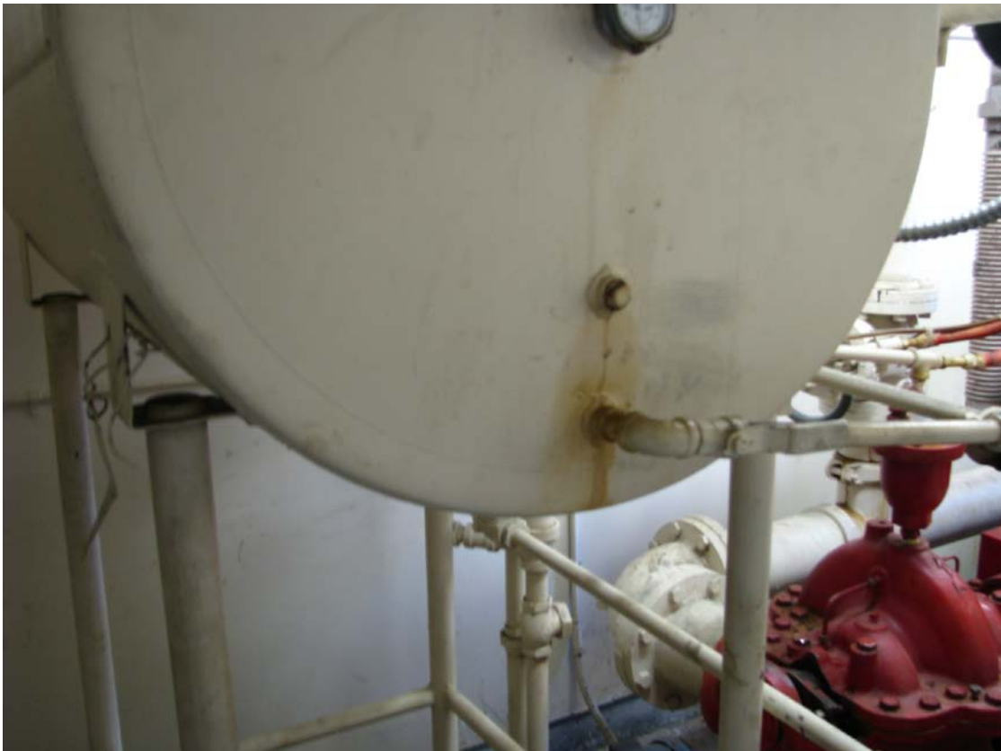
Tanks A-18-5 – Bldg 400
