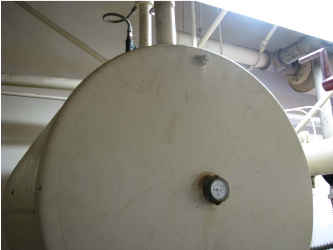
Tanks A-18-5 – Bldg 400
