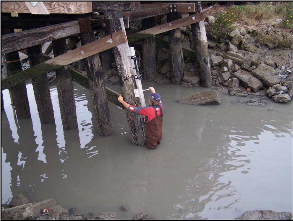
Figure 1. Macro Tide installation at Meeker Slough on 11/16/2006.
