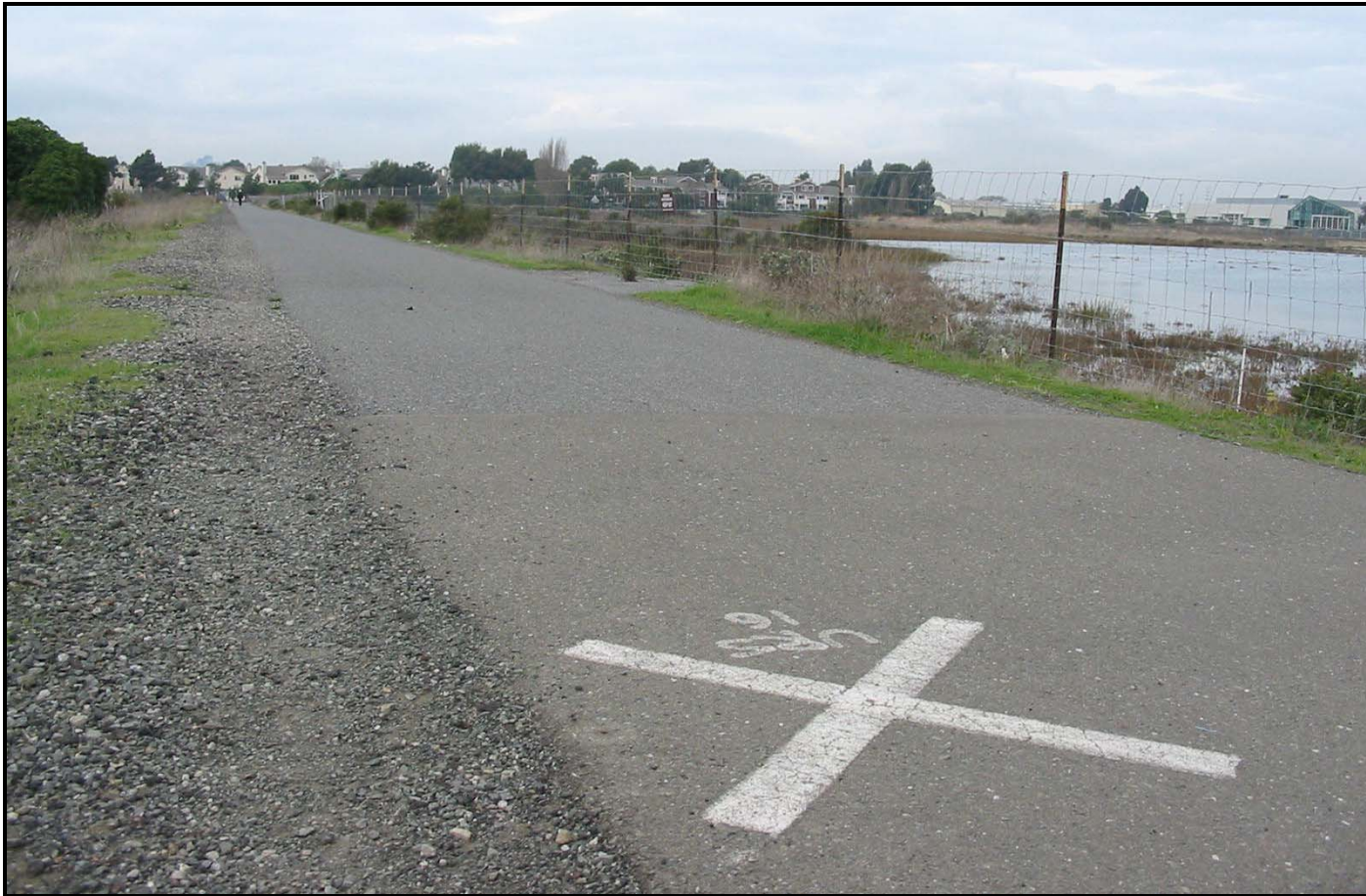
Figure A.11. Existing survey control point located on the EBRPD Bay Trail at the southeastern corner of the project site. The coordinates of the control point were confirmed with 2004 surveyed coordinates. This location was used as a control point in the November, 2006, and August, 2007 surveys. Photo dated 11/21/2006.
