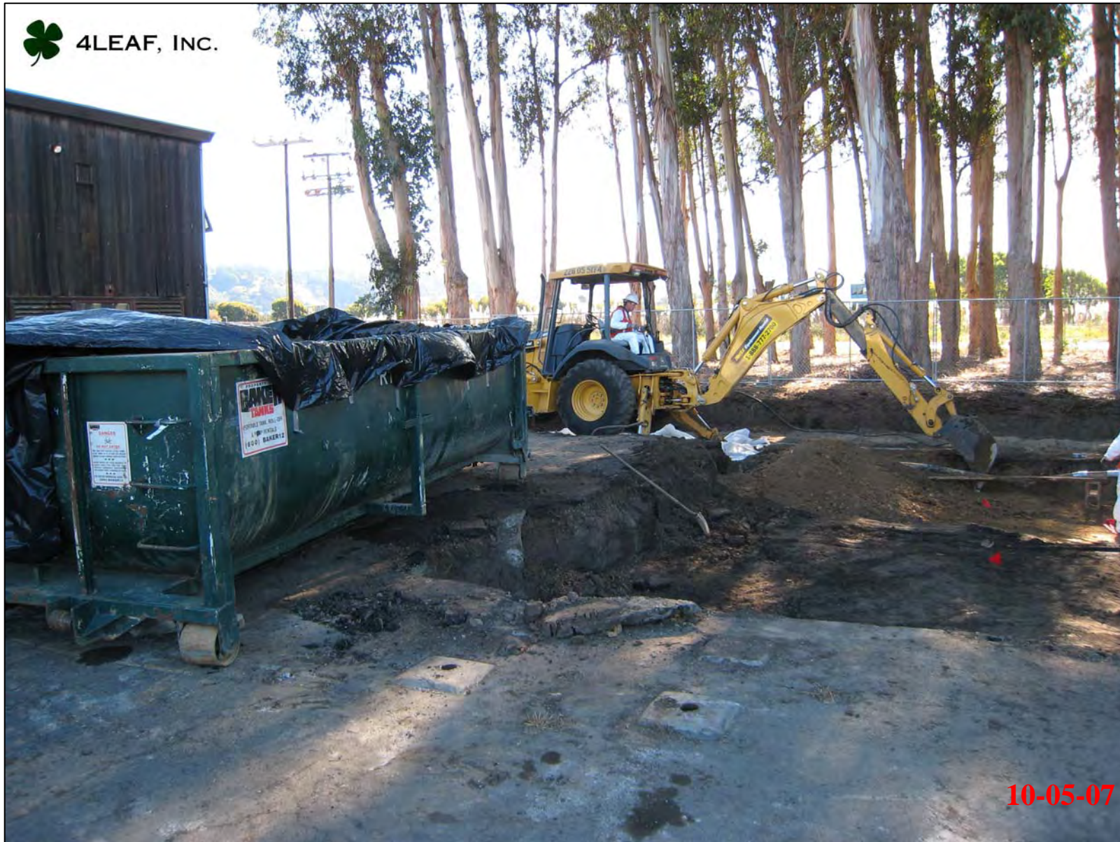
View of area of 3 ½-ft cut in excavation.
