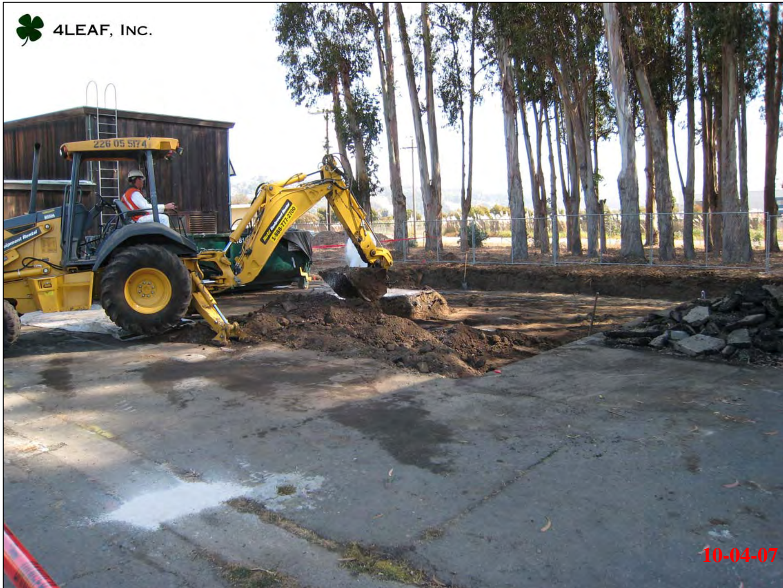
View of excavation. View looking northeast.
