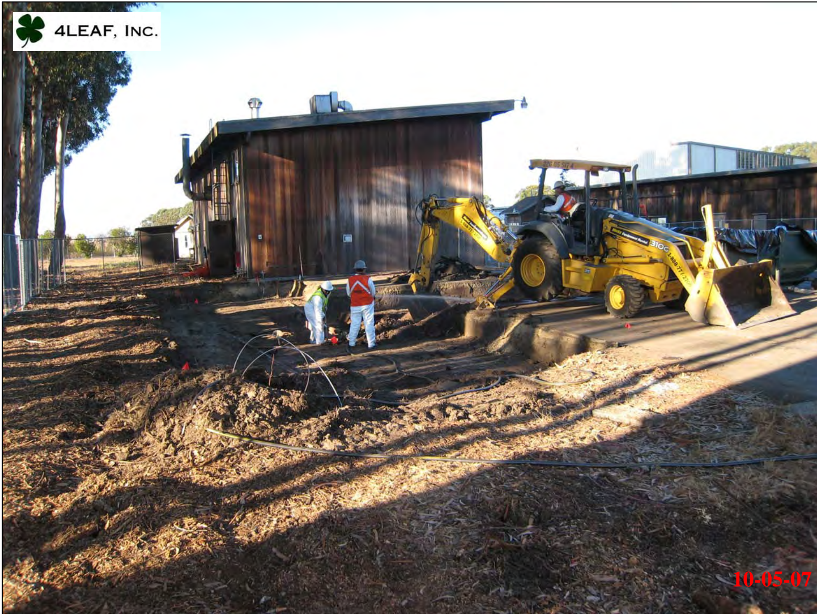
View of excavation activities. View looking south towards Bldg. 472.
