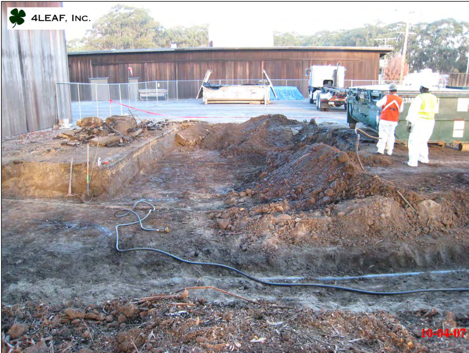
View of excavation looking west towards Bldg. 473.
