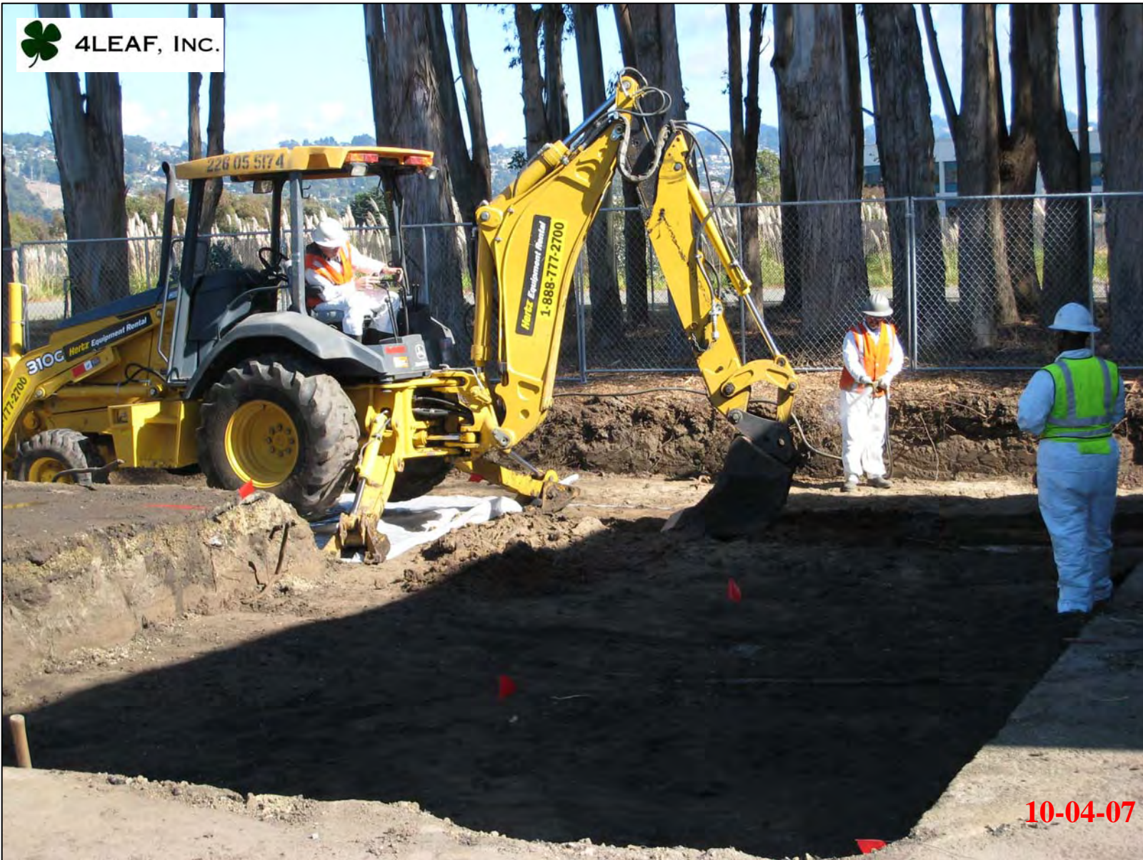
Excavating for 3 ½-ft cut along along site utilities.
