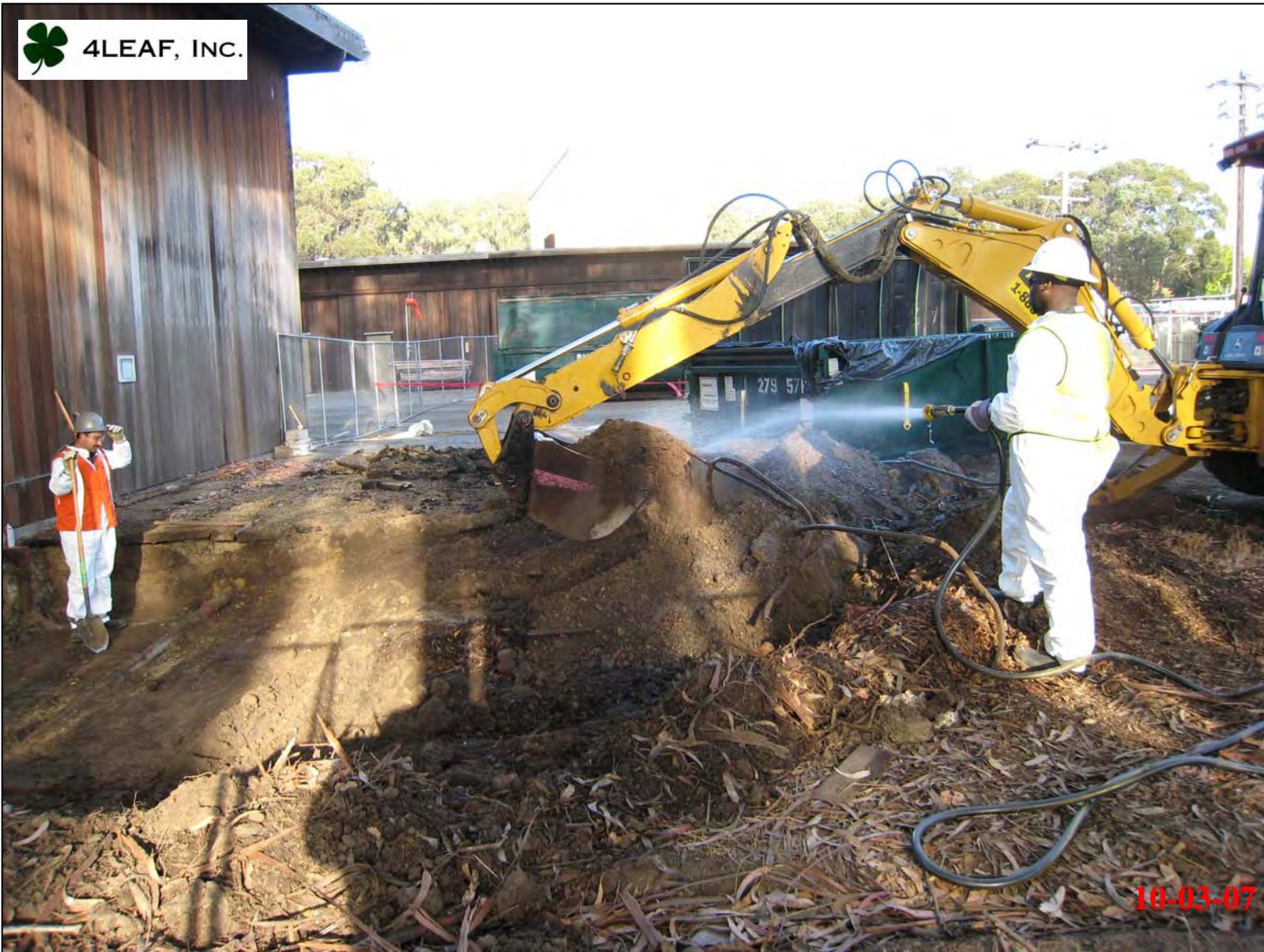
Applying dust suppression during excavation activities.
