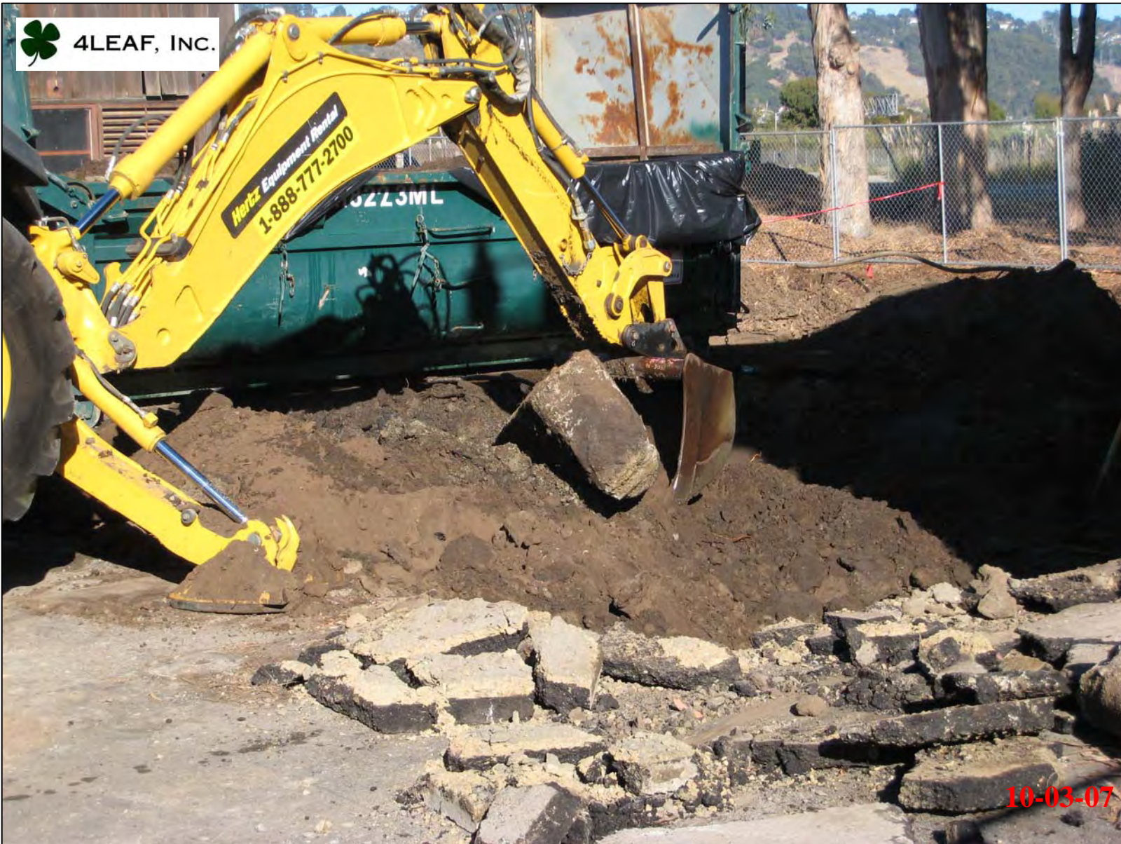
Concrete footings being removed from beneath former concrete pad.
