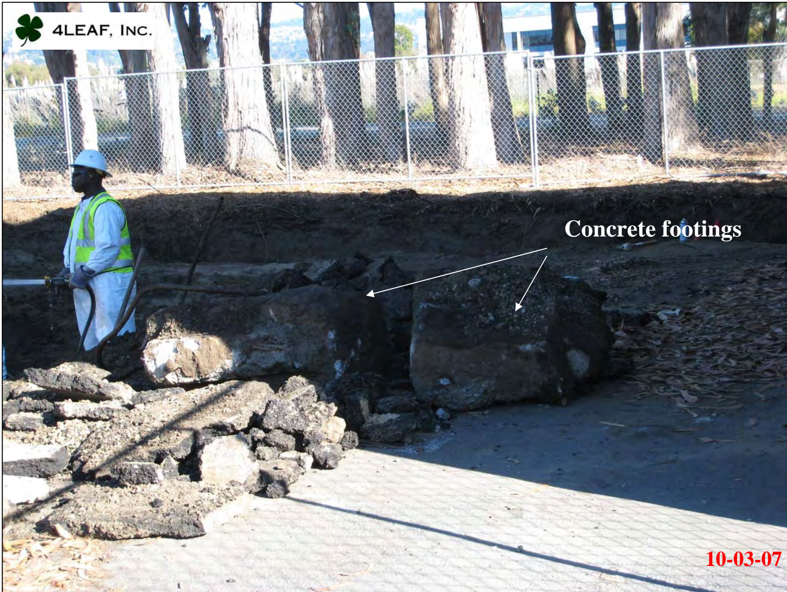
Concrete footings removed from beneath former concrete pad.
