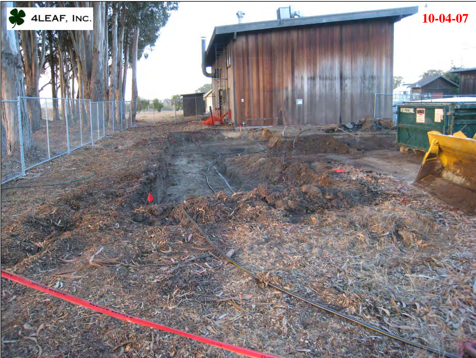
View of excavation looking south towards Bldg. 472.
