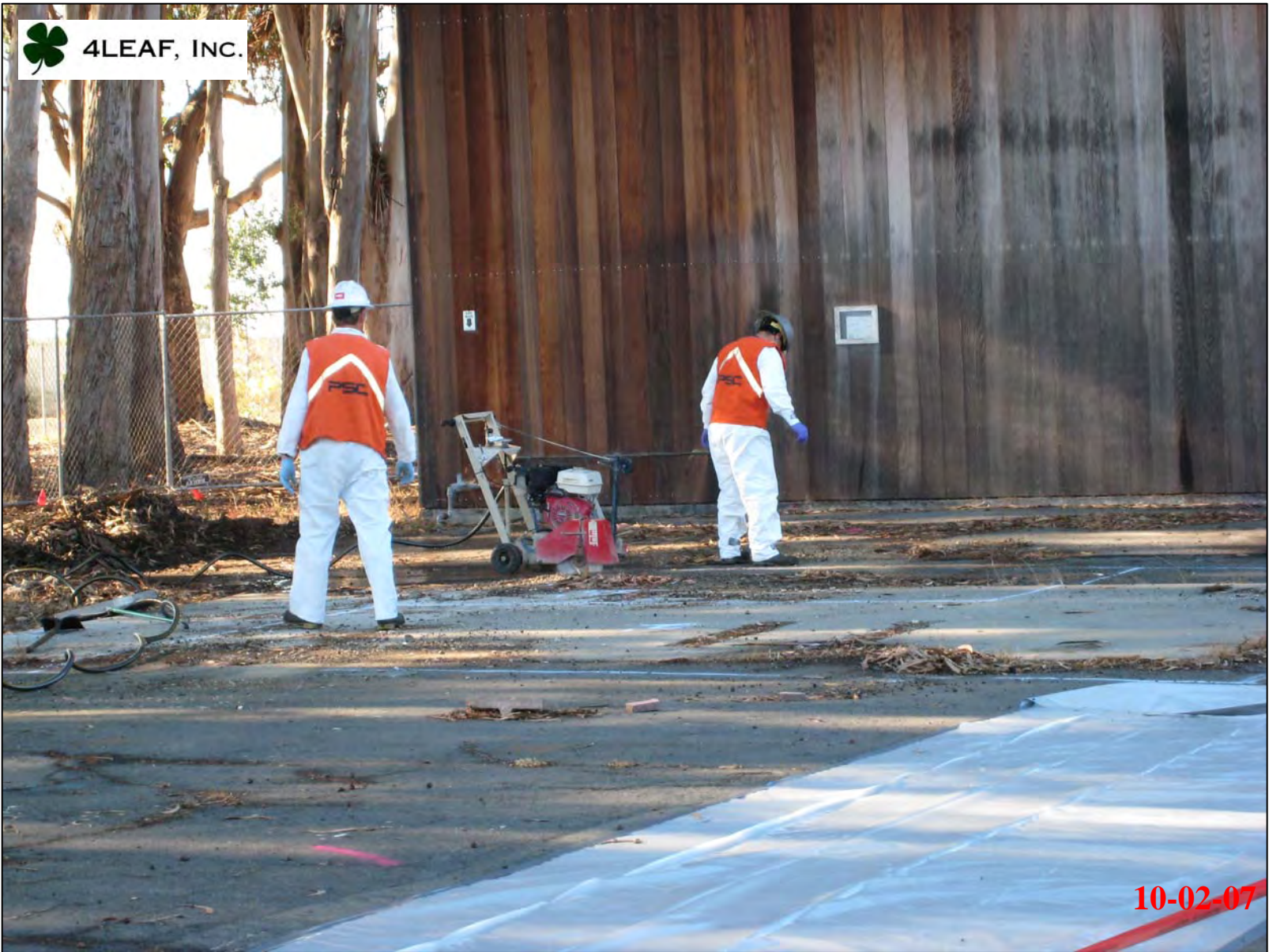
Saw cutting concrete pad and asphalt over excavation area.
