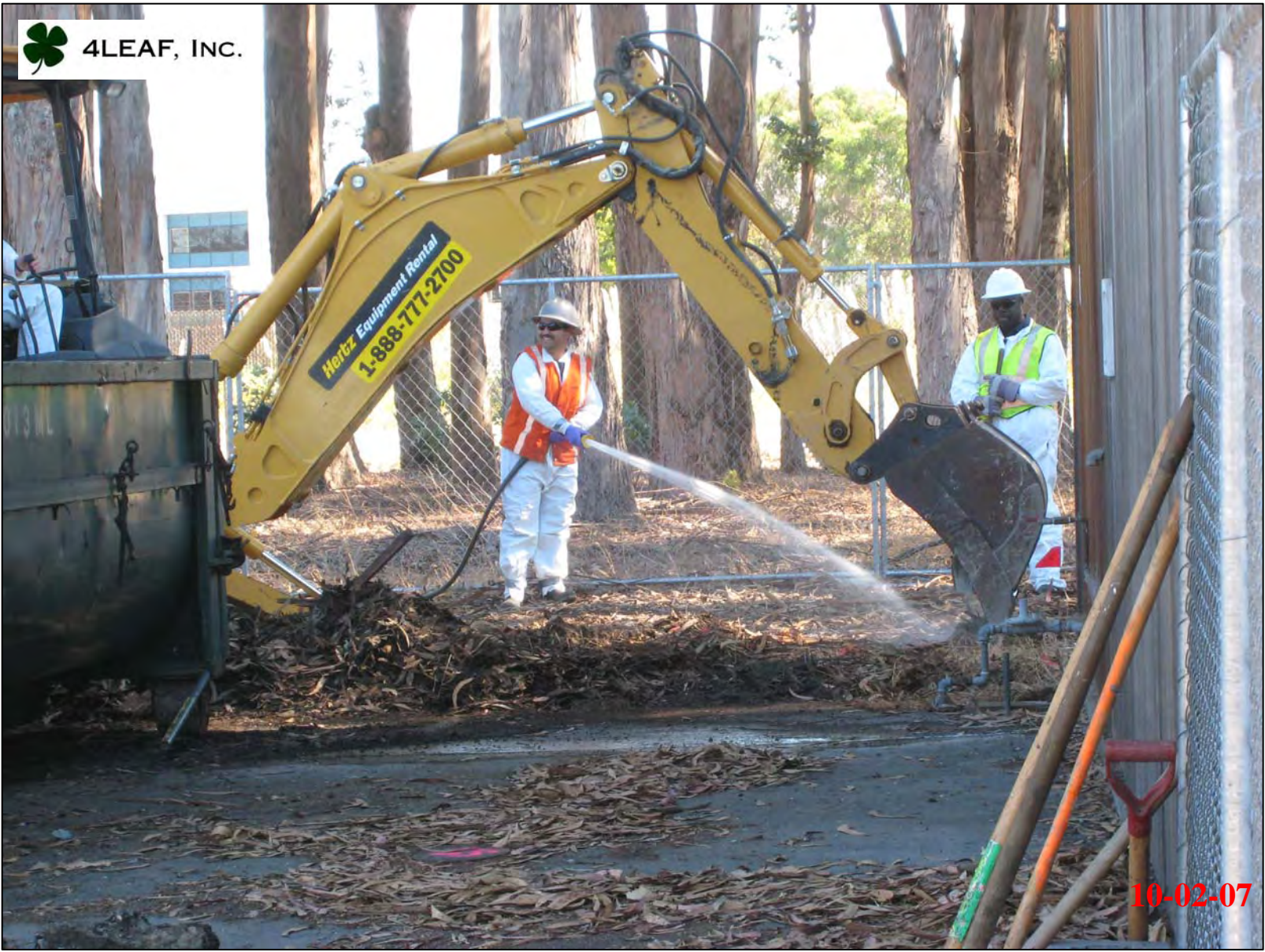
Using dust suppression as excavation begins along northeast corner of Bldg. 472.
