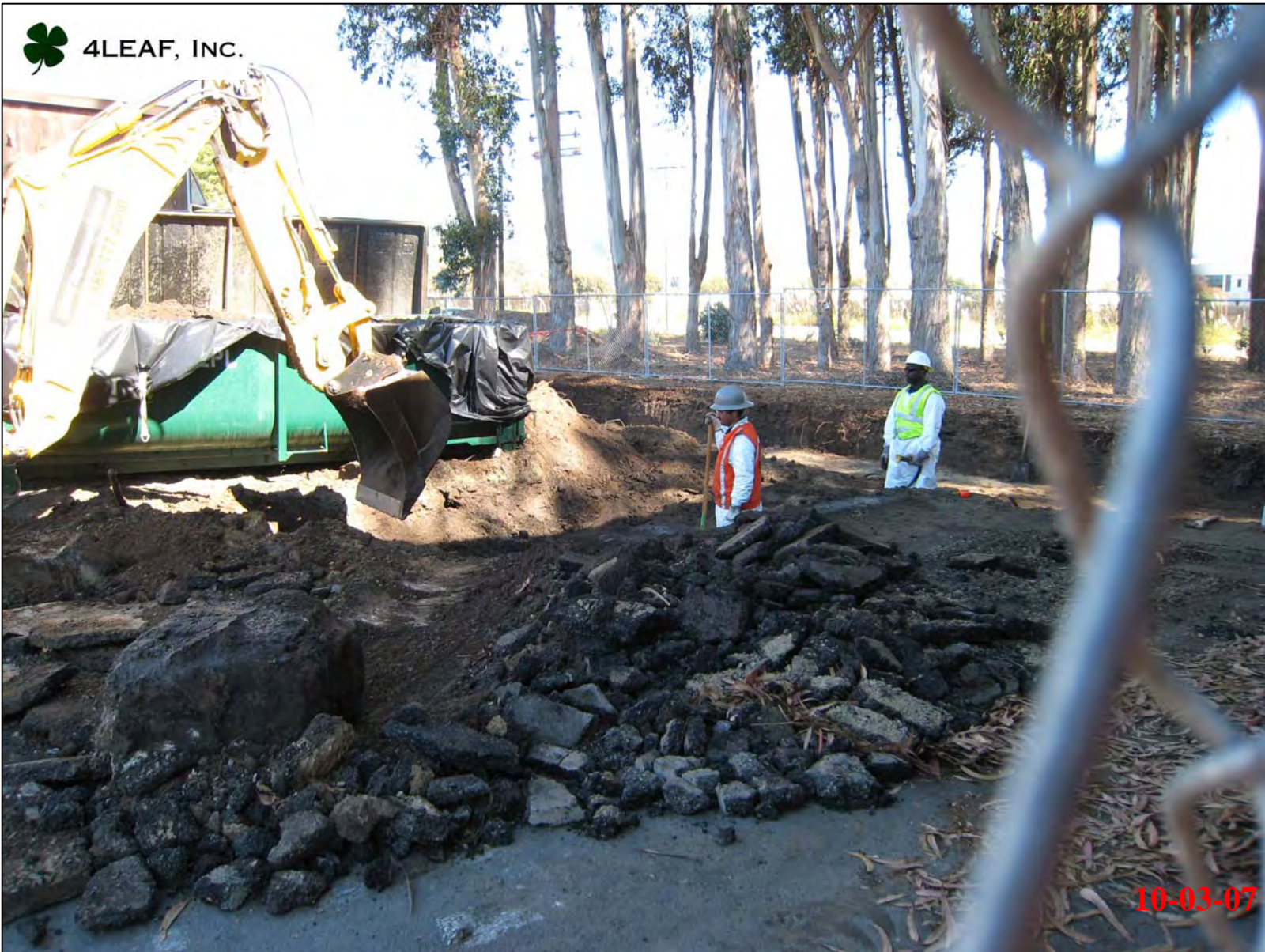
View of excavation area (2-ft cut).
