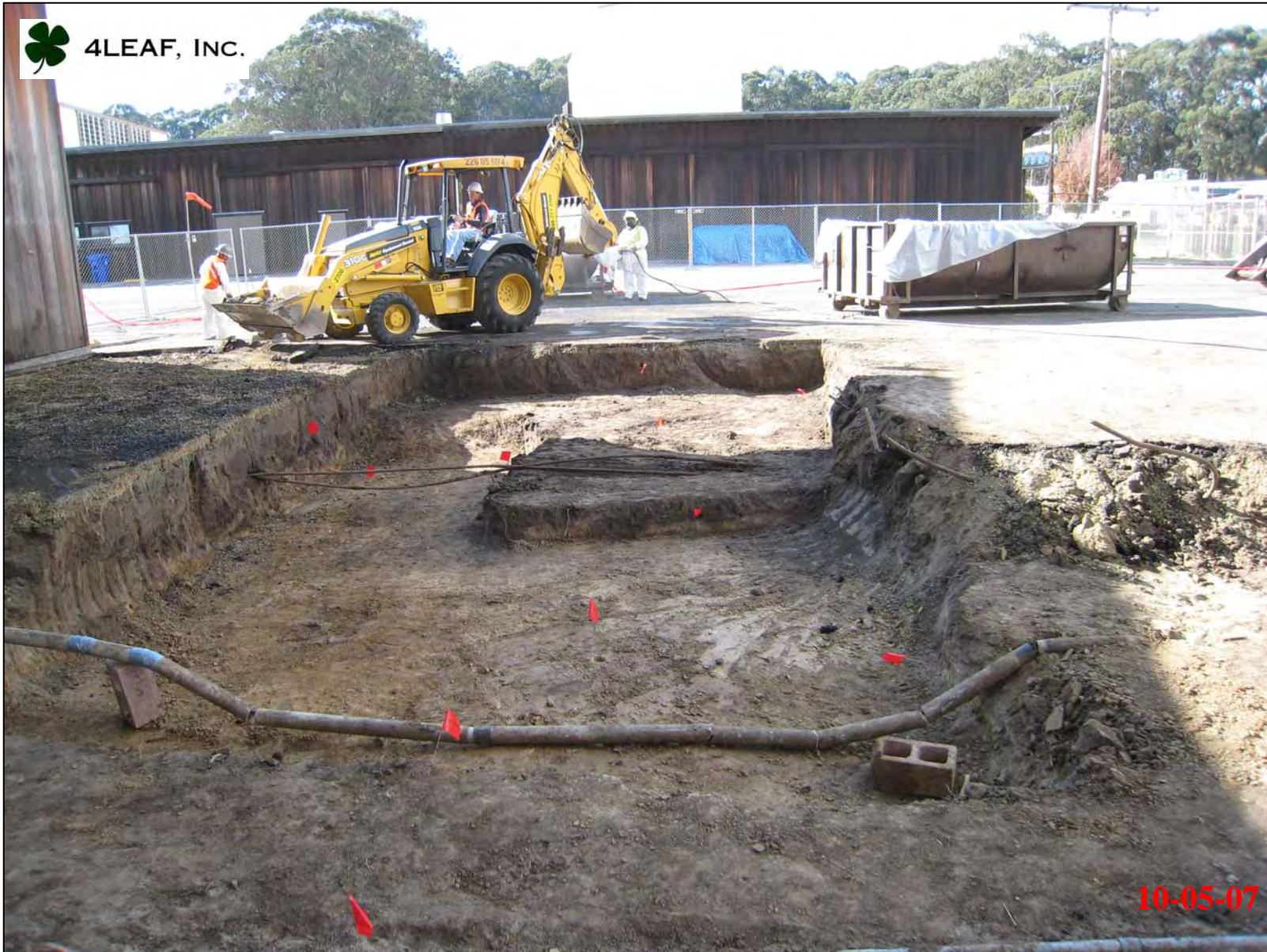
View of excavation after soil confirmation samples collected.
