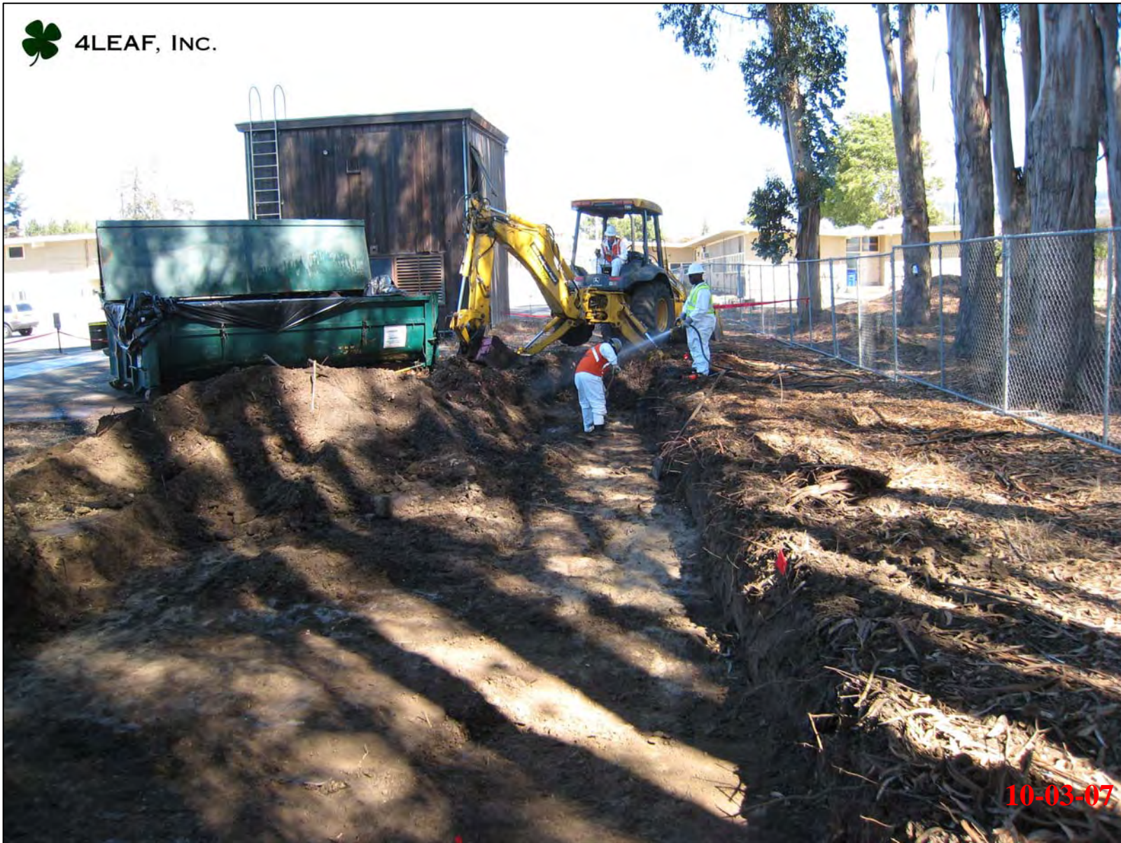
View of excavation (looking north towards Bldg. 476).
