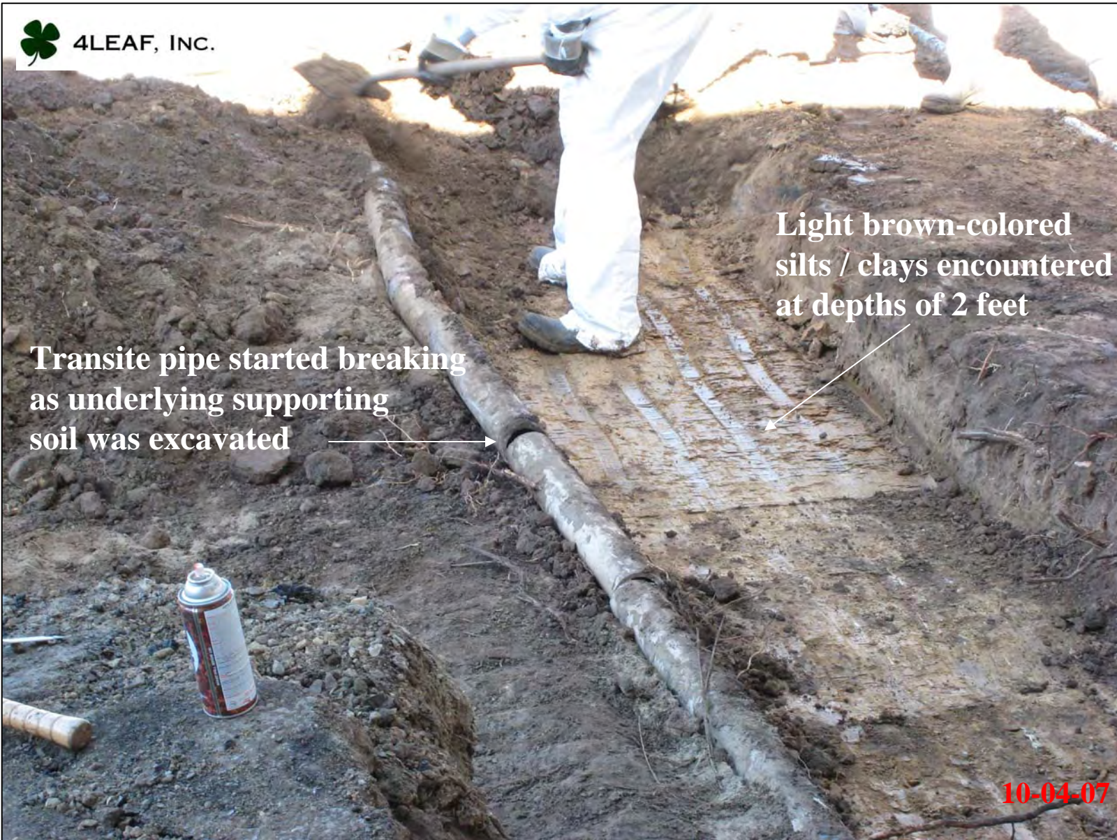
View of broken conduit for electrical line into Building 472.
