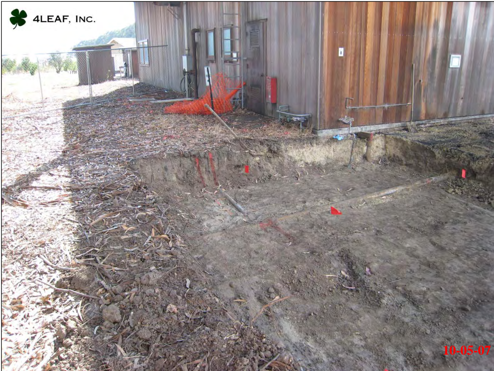
View of excavation after soil confirmation samples. View looking towards Bldg. 472.
