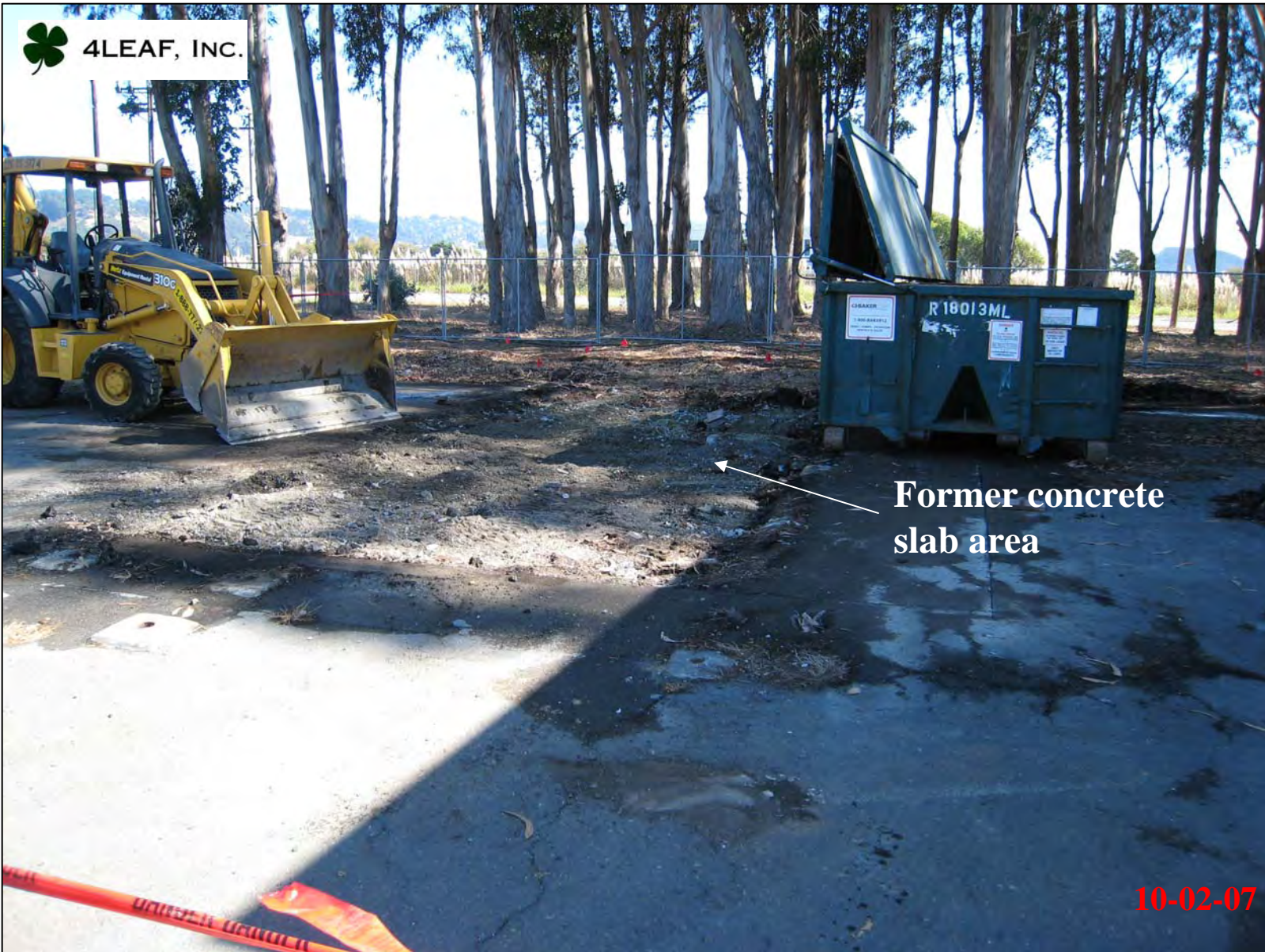
View of excavation after concrete slab removed.
