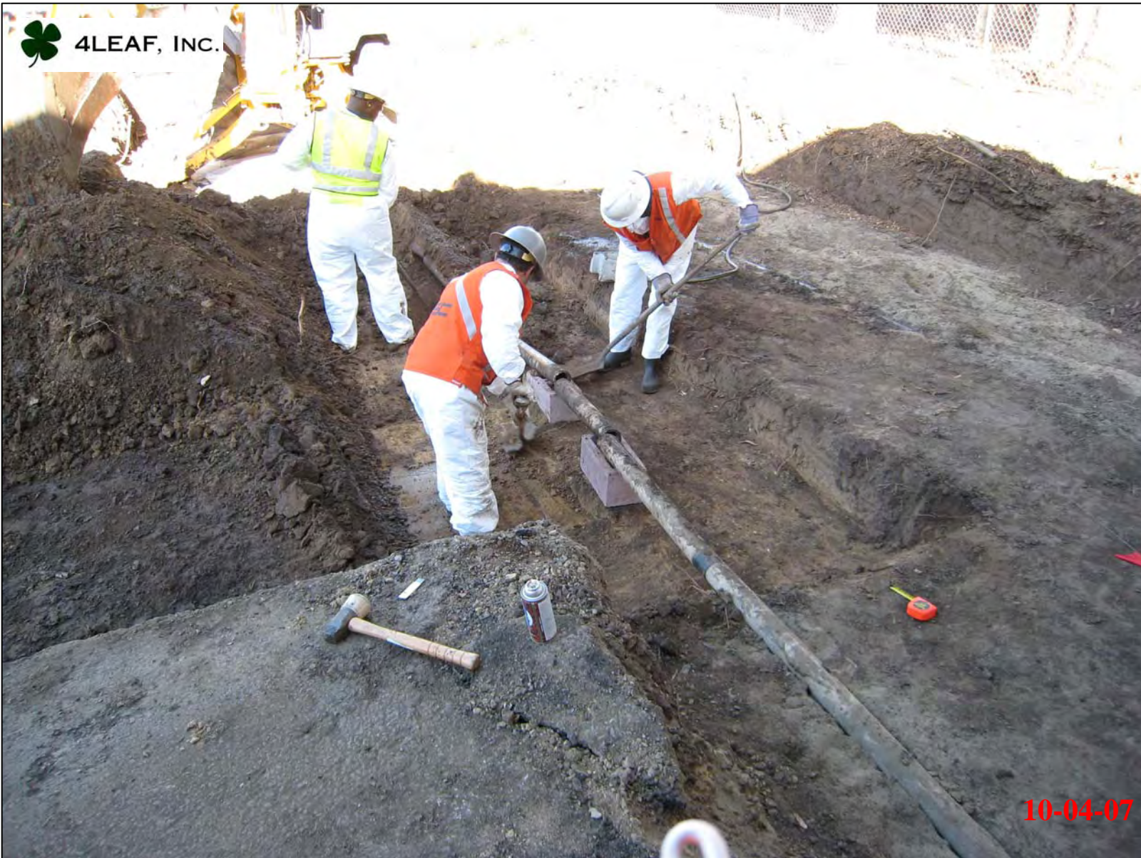
Electrical conduit was supported using blocks after underlying soil was hand excavated.
