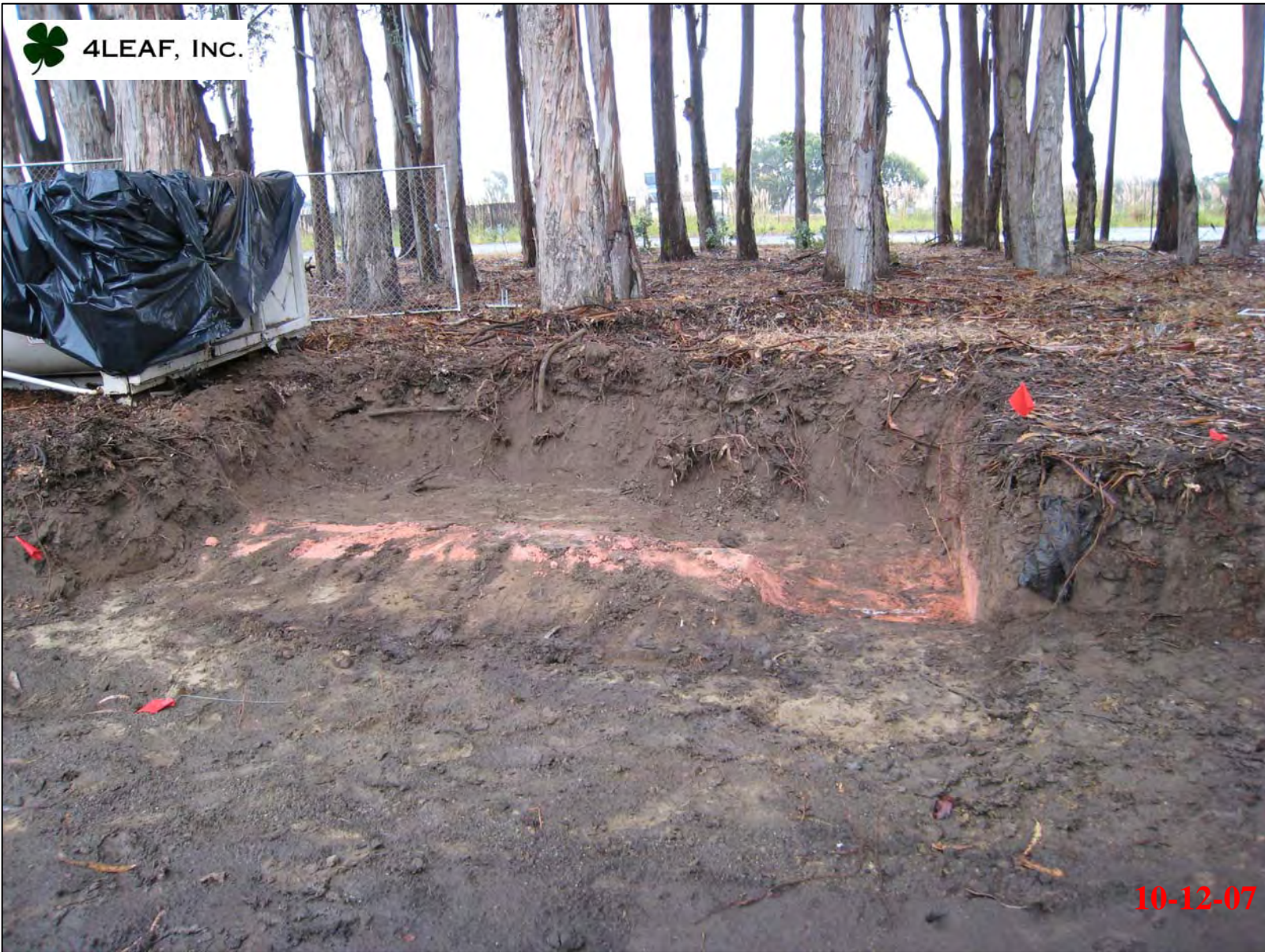
View of completed over-excavation area.
