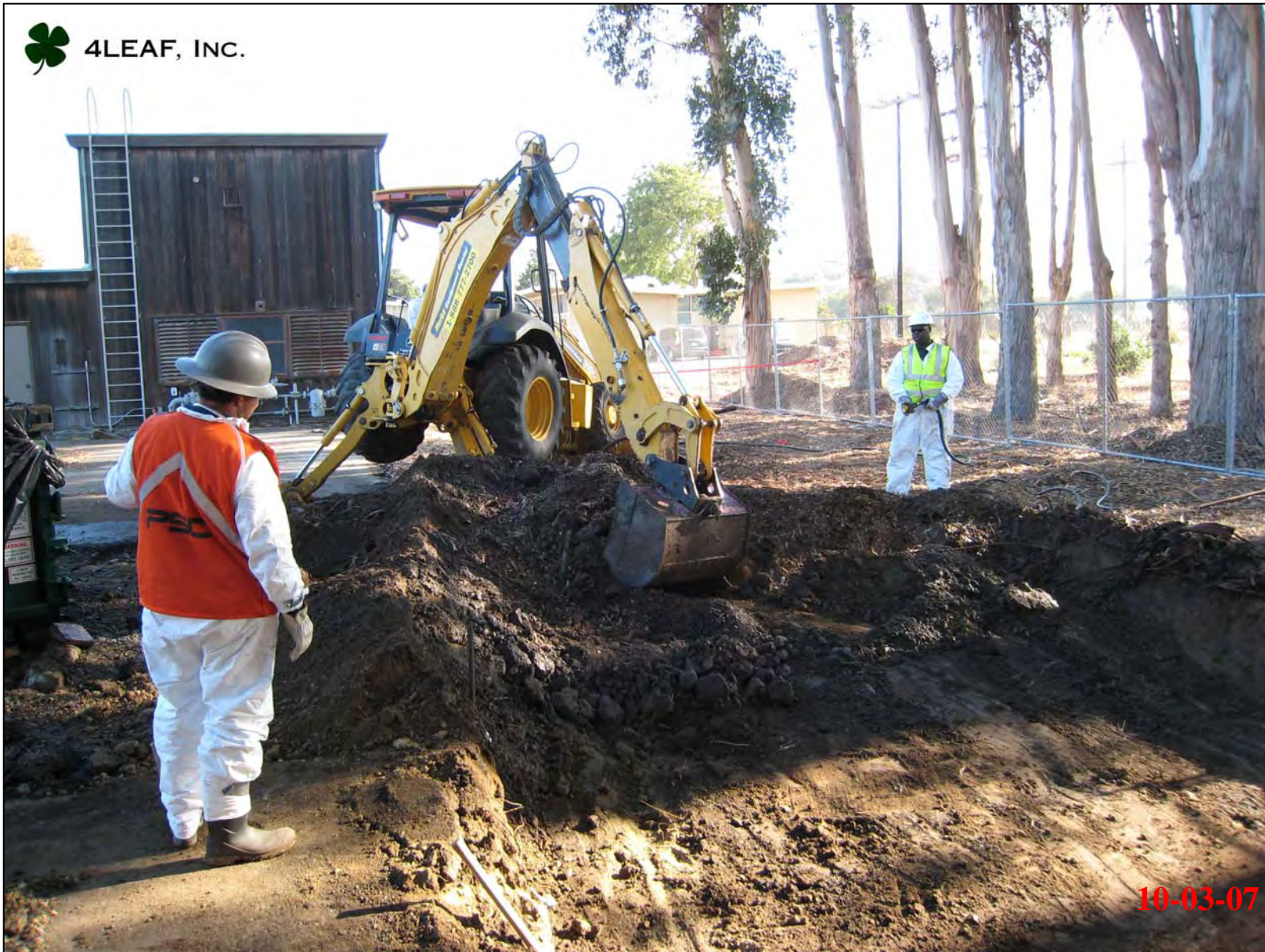
View of excavation (looking north towards Bldg. 476).
