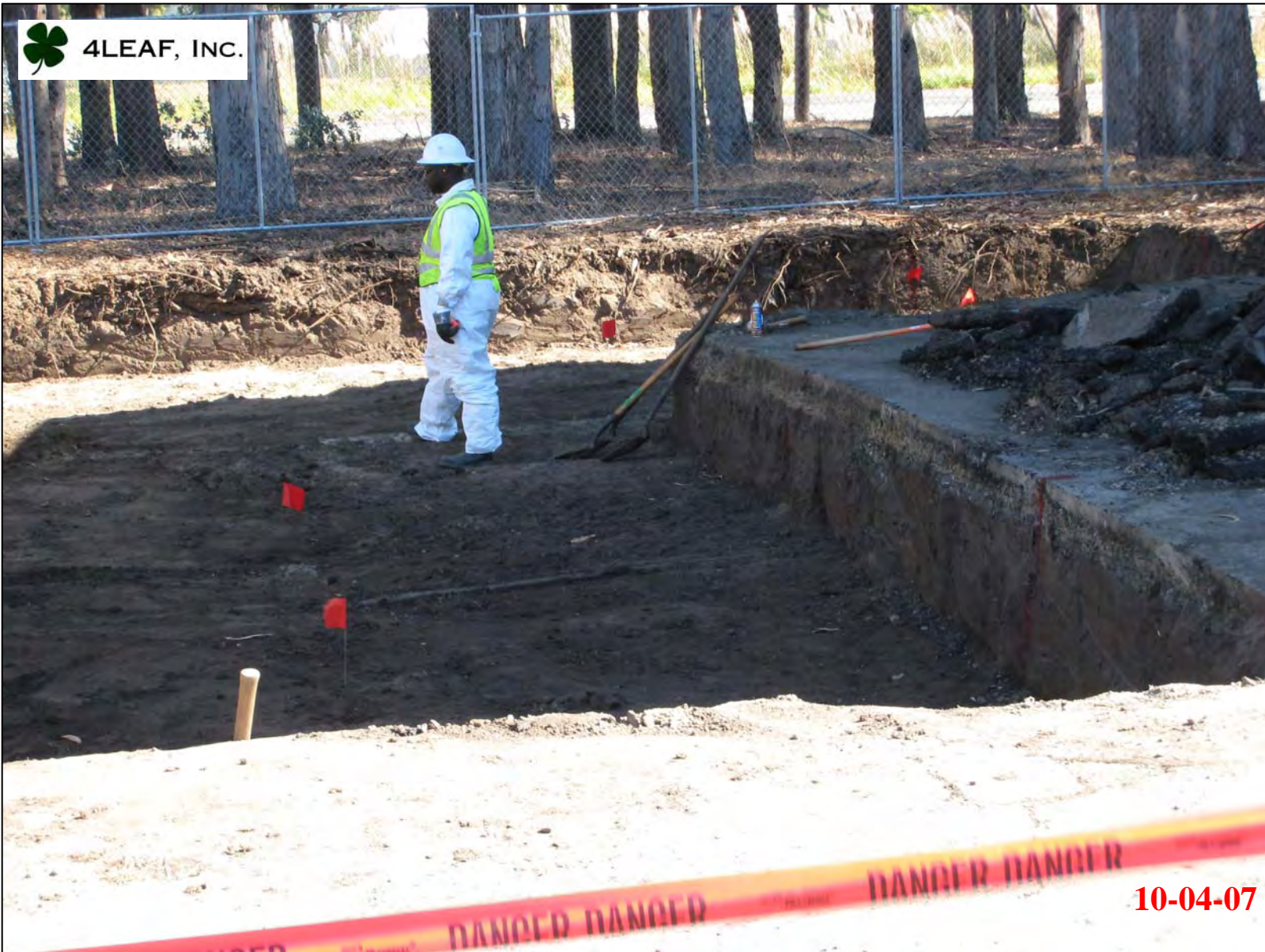
View of excavation in area of 2-ft cut.
