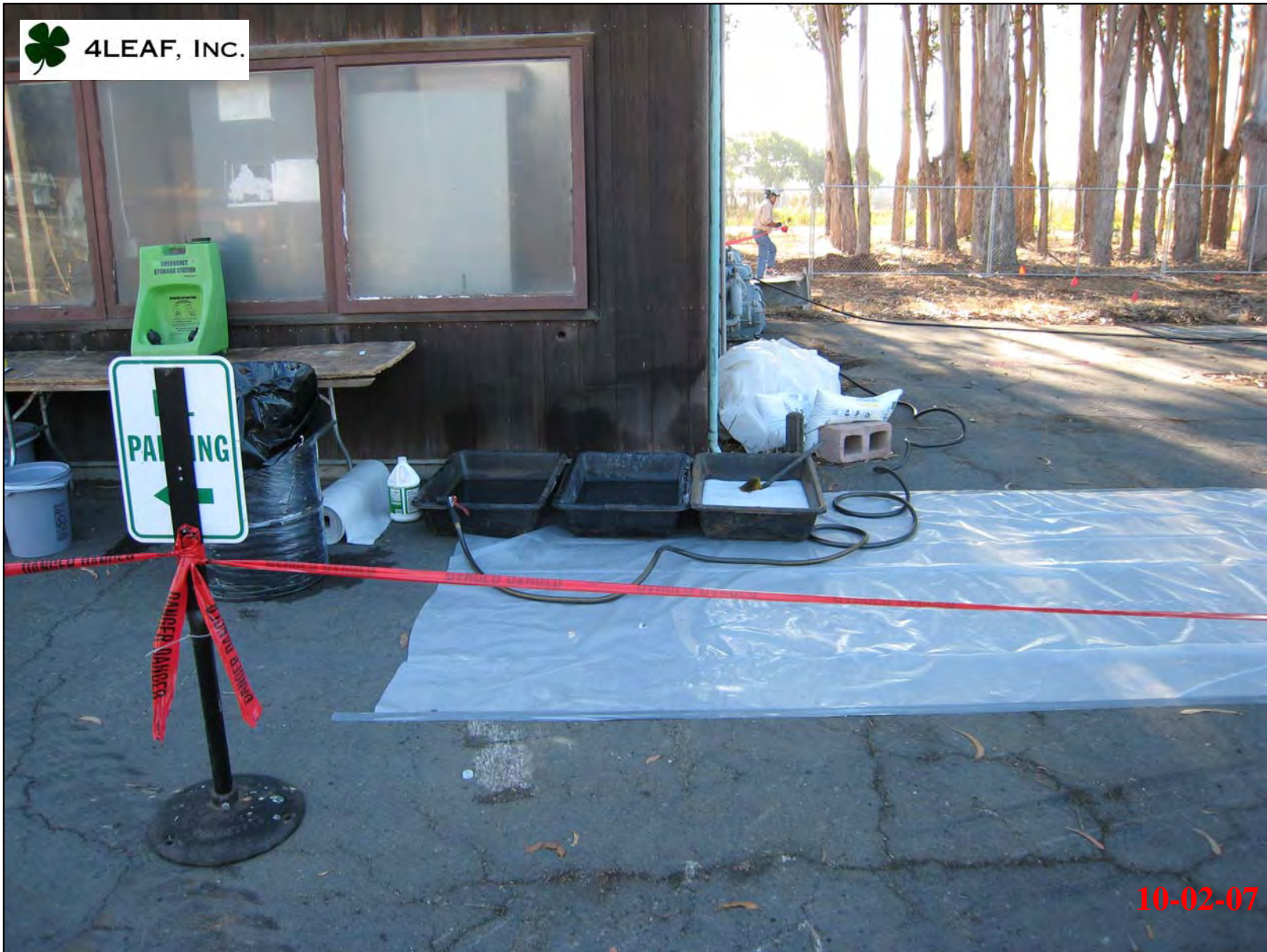
PSC's decon station set up adjacent to Building 476.
