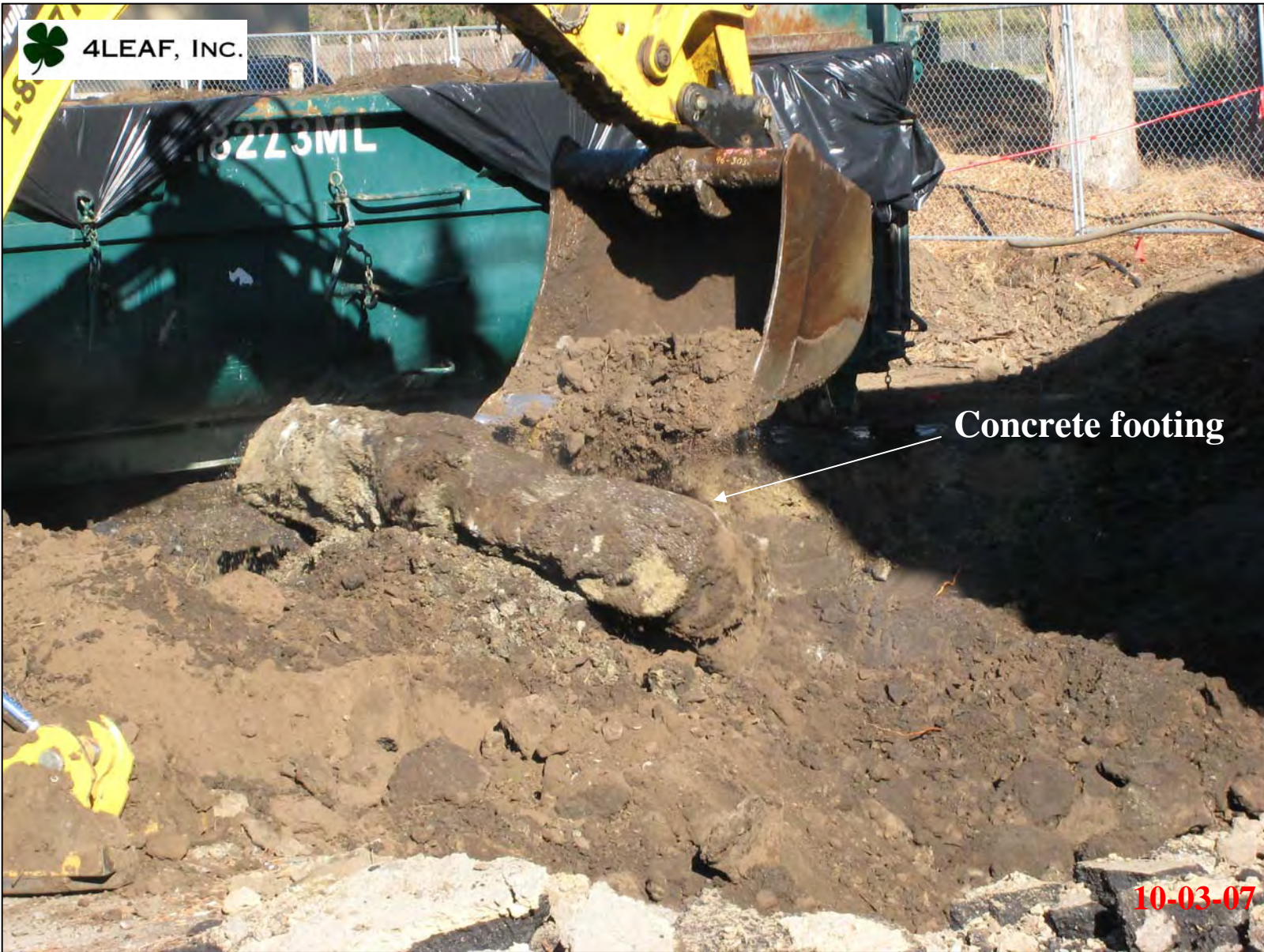
Removing concrete footings.
