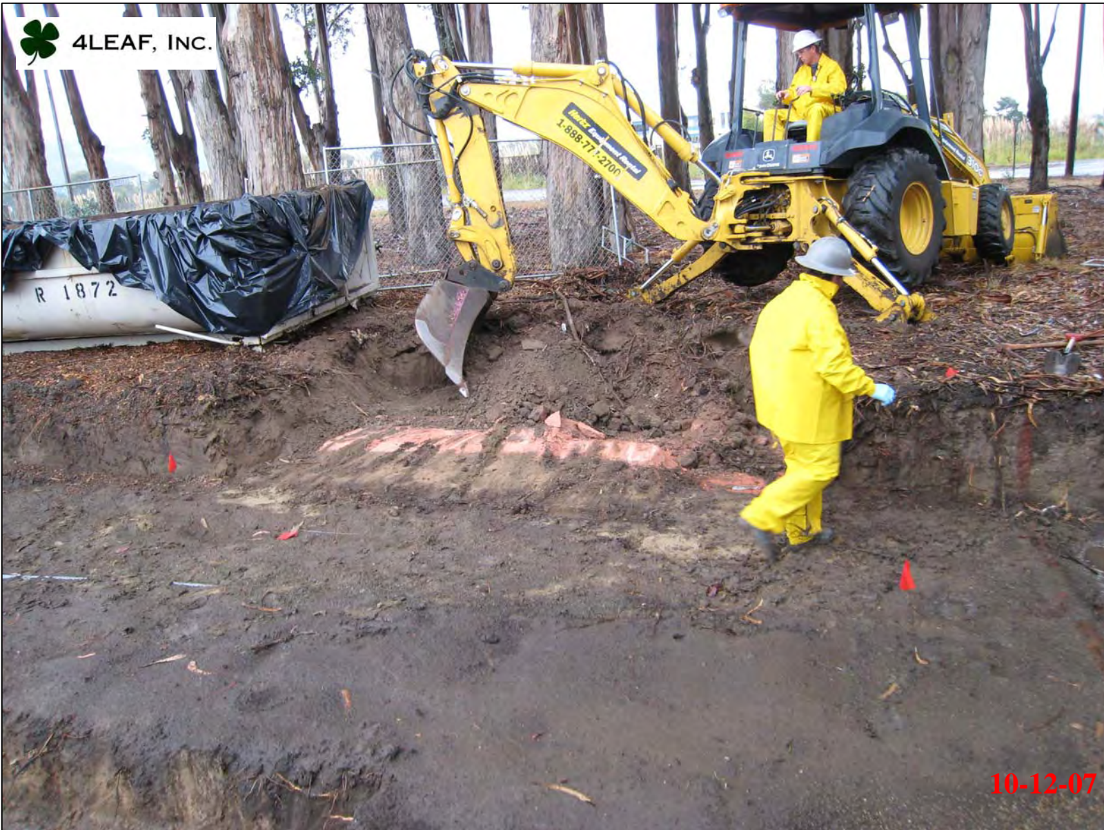
Performing over excavation activities.
