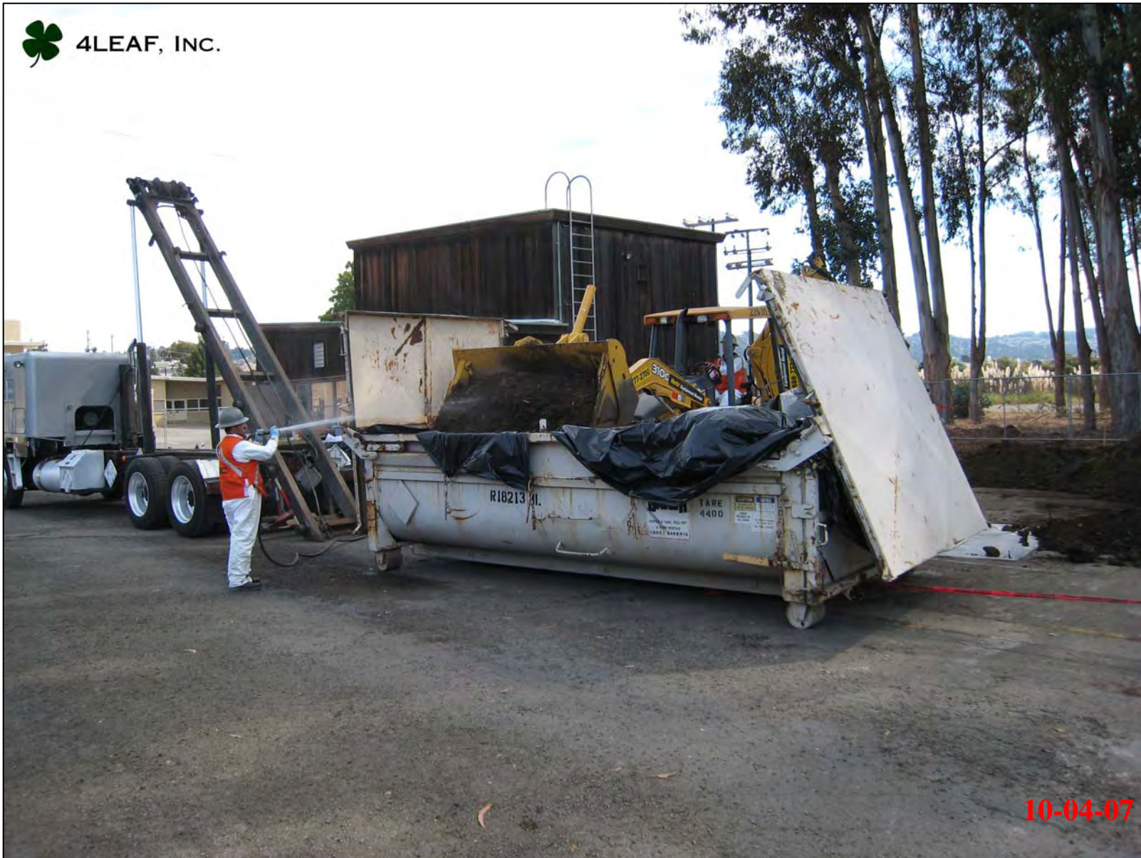
Using dust suppression while loading soil into bin.
