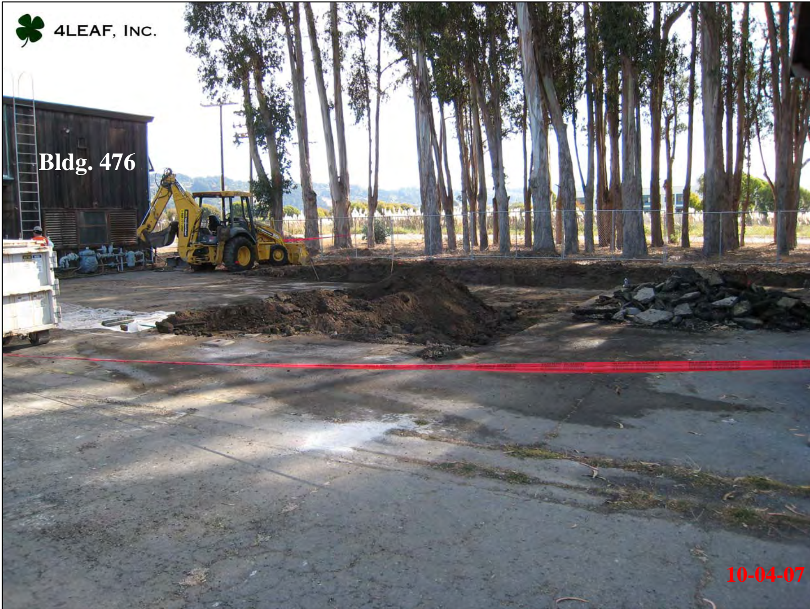
View of excavation. View looking northeast.
