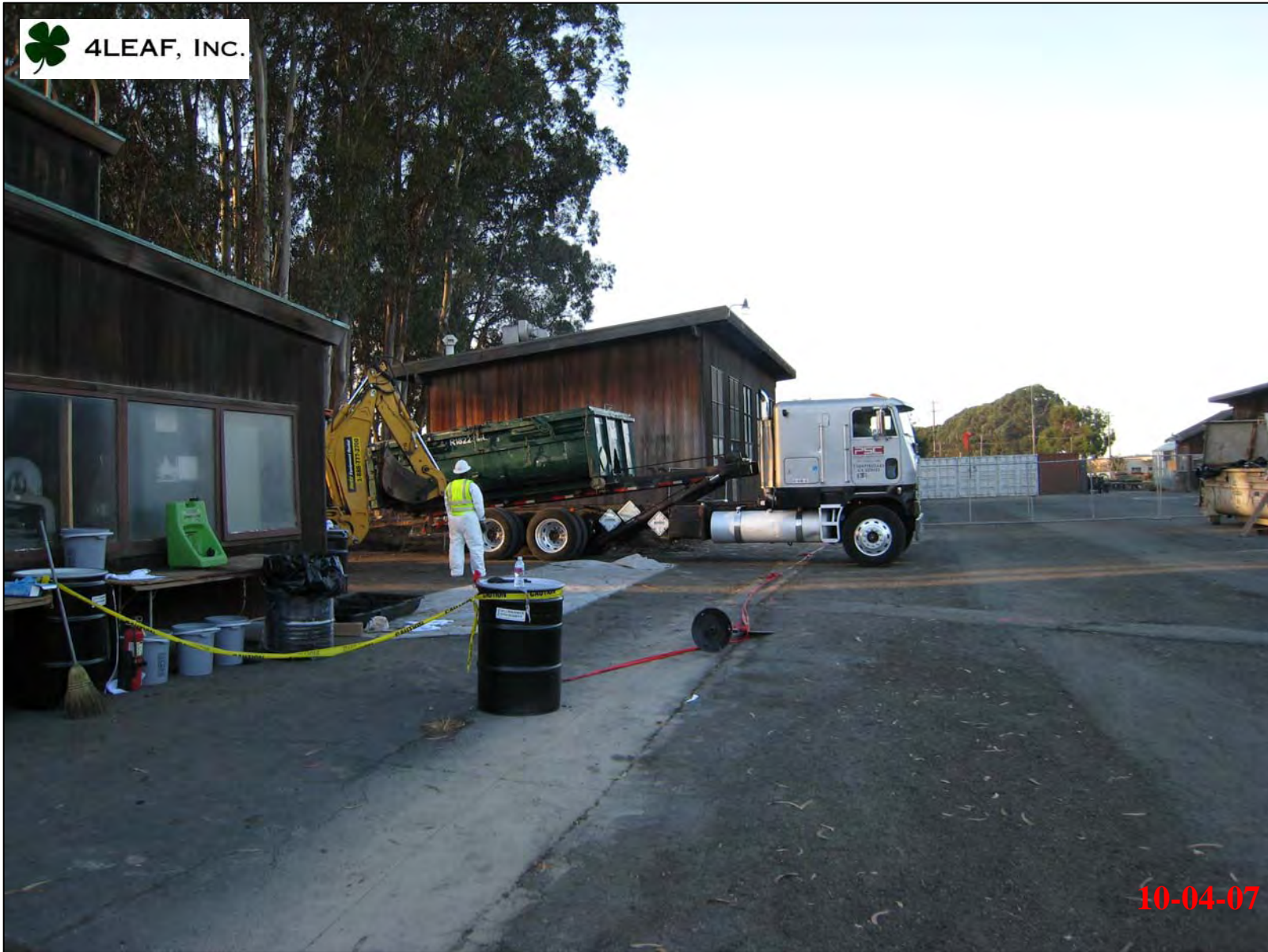
Loading out soil bin for transport to fenced area by Bldg. 102.
