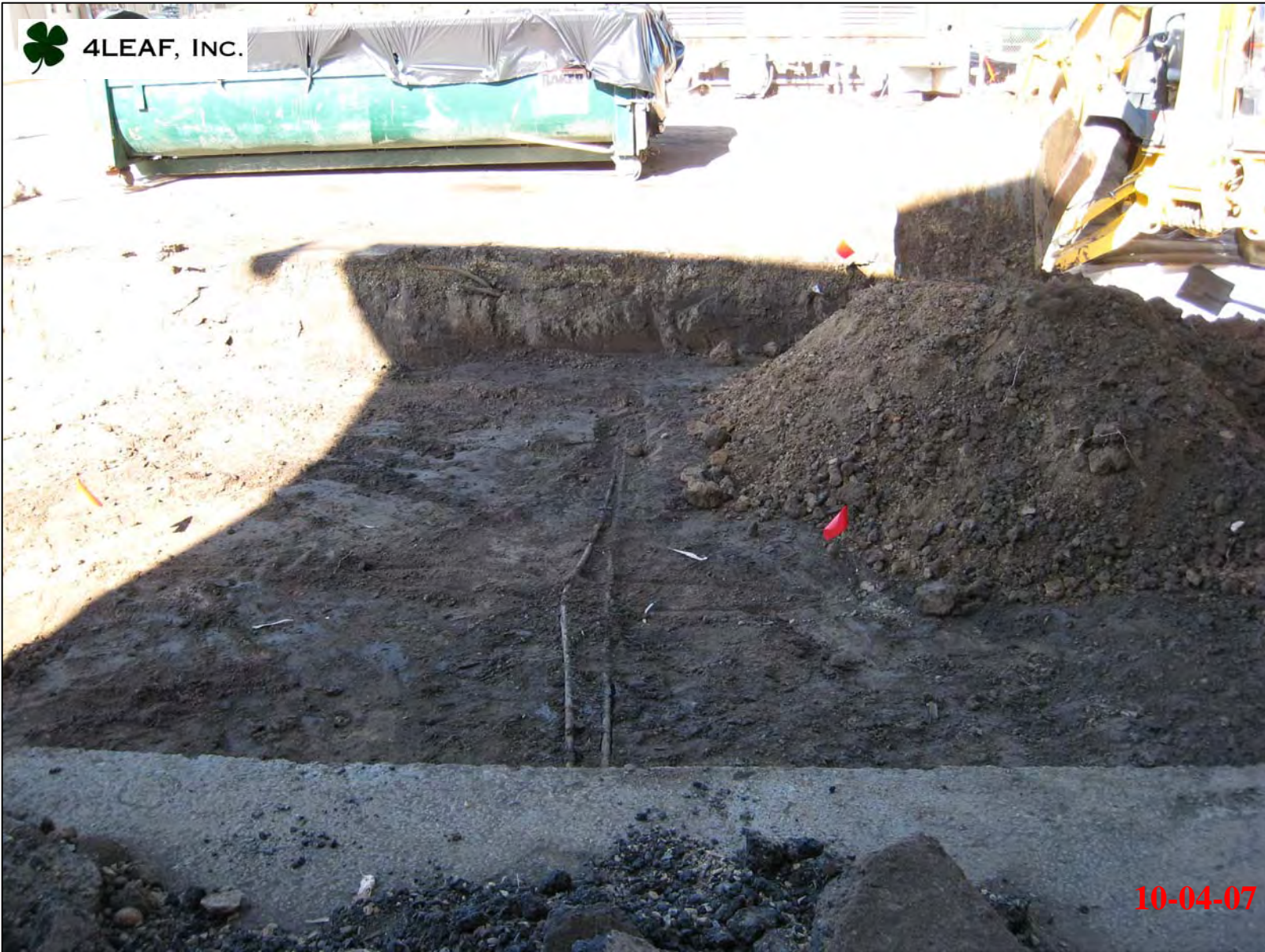
Miscellaneous utilities encountered in excavation. View looking west
