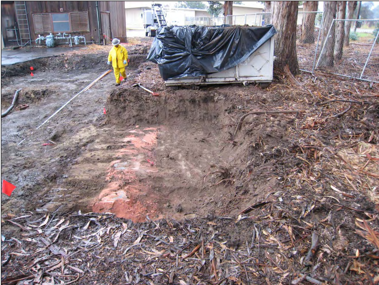
View of completed over-excavation area.
