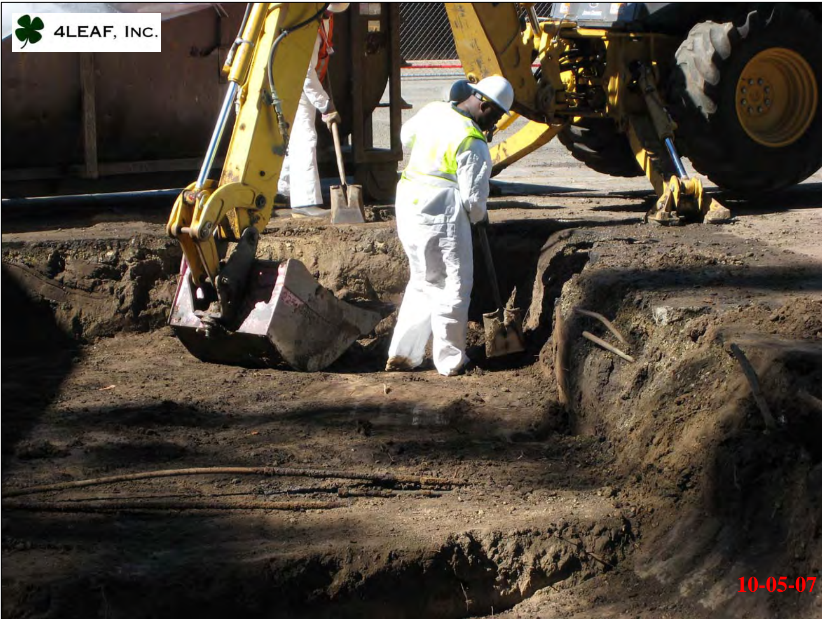
Using shovels to clean up final amounts of loose soil from excavation.
