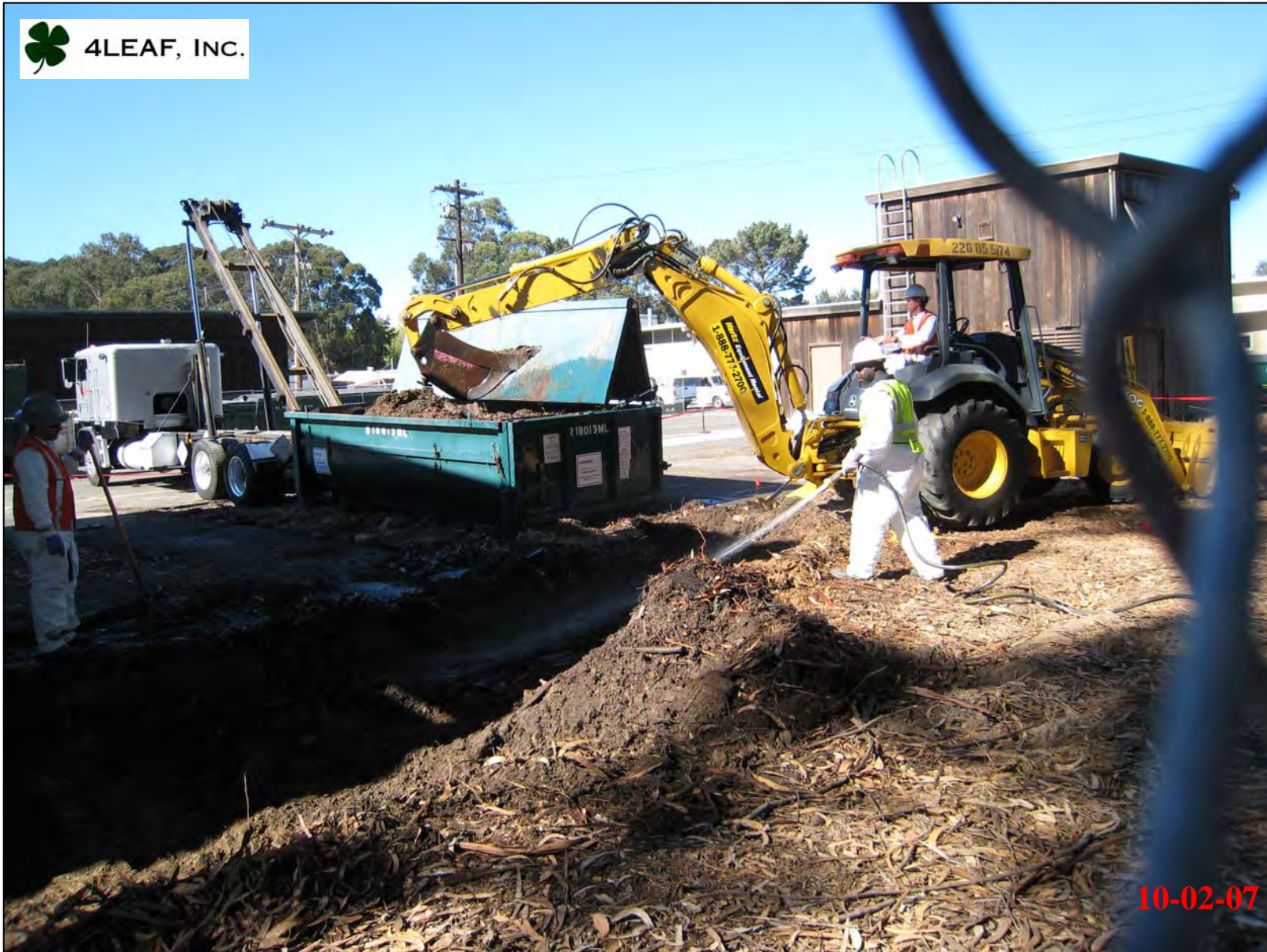
View of excavation along northeastern corner of Bldg. 472.
