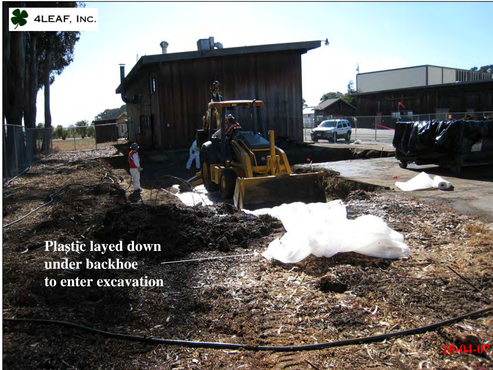
Backhoe in excavation to excavate for 3 ½-ft cut along location of utilities.
