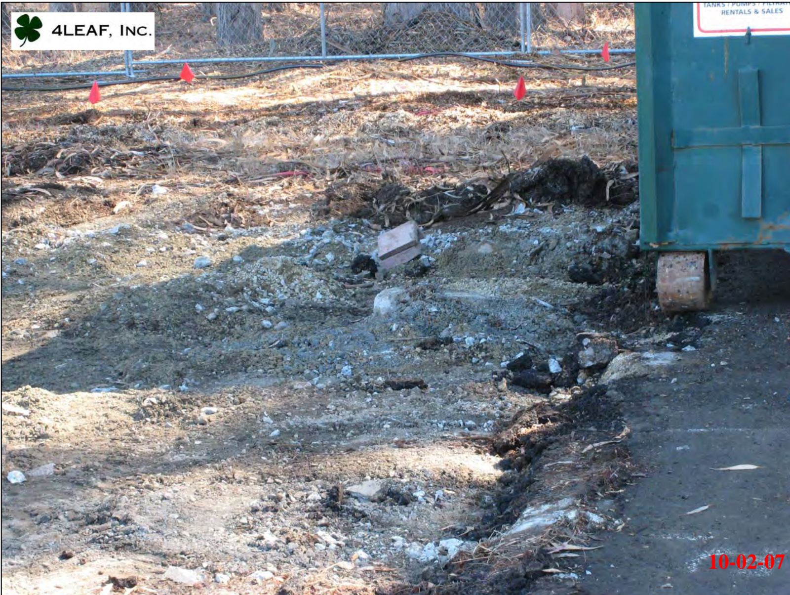
View of excavation after concrete slab removed.
