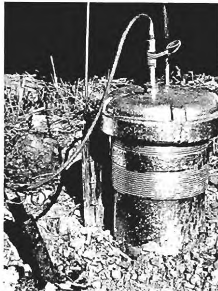
FIGURE 5b. Sampling well head with piezometer and sampling tubes
