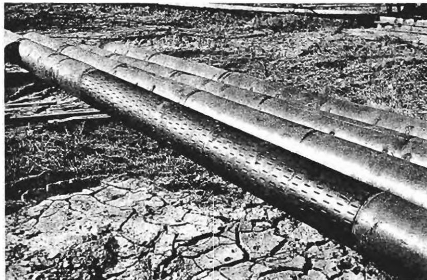
FIGURE 2. Recharge well screen and casing
