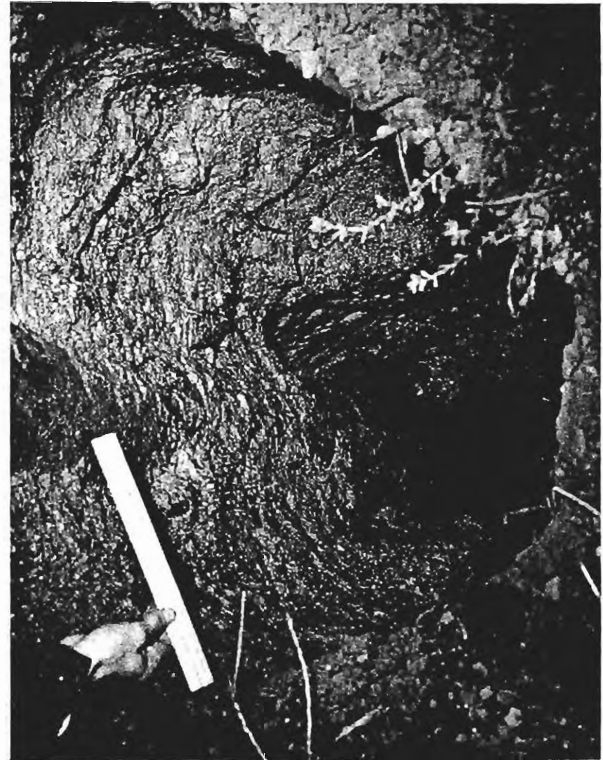
FIGURE 31. Cave-in at original recharge well
