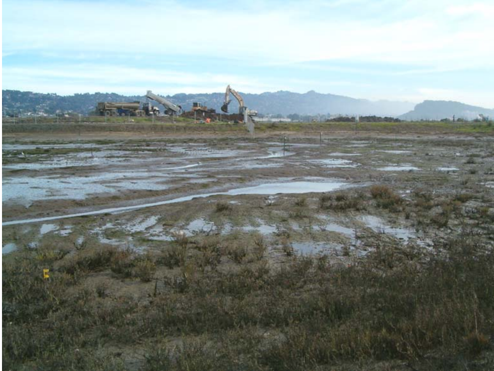
Photodocumentation Location 5 – photograph taken facing east
